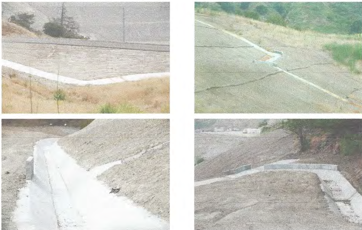
Photo 10: Drainage works on graded slope below Flare 3
