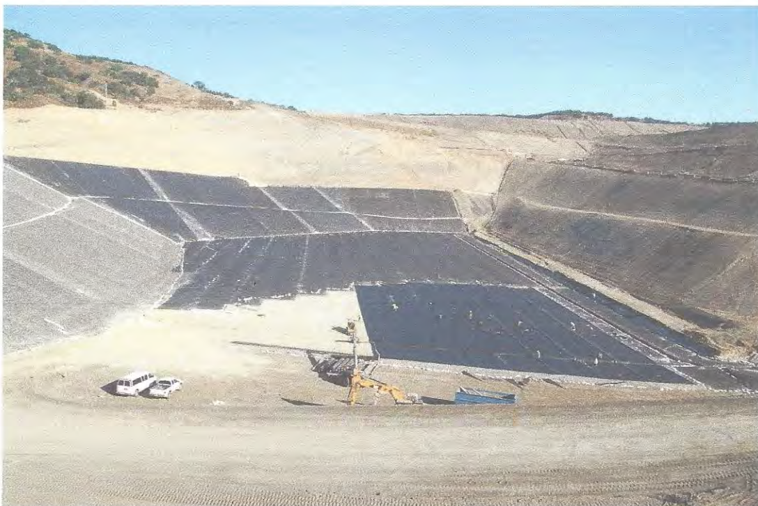
Photo 16: Deployment of 80 mil geomembrane on top of 2ft-thick clay layer at Cell CC4 Phase 4
