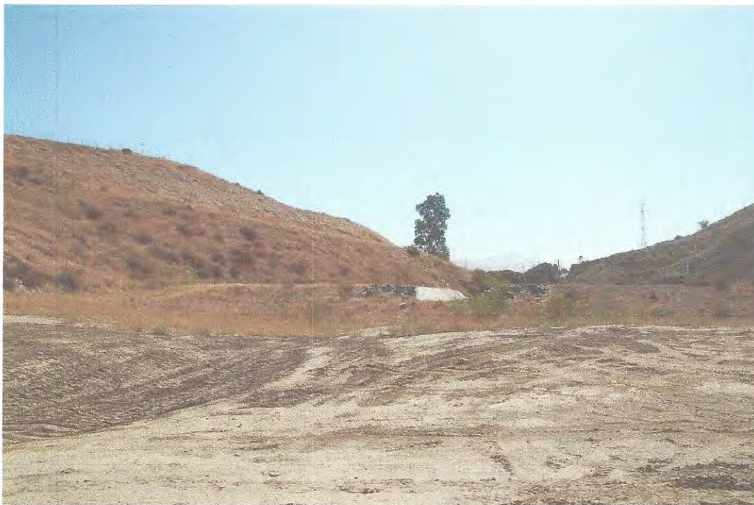
Photo 6: Regraded erosion gully at basin at toe of Cell CC#
