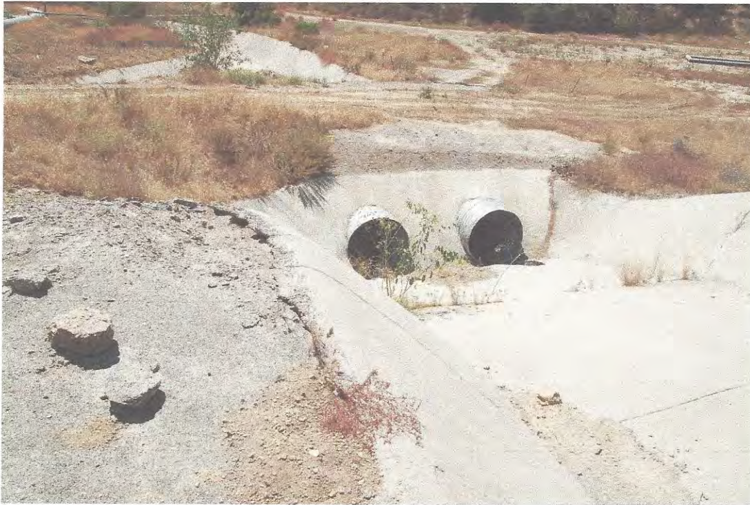
Photo 9: Erosion at contact between shotcrete of spillway and vegetation growing in spillway at southern half of Basin D
