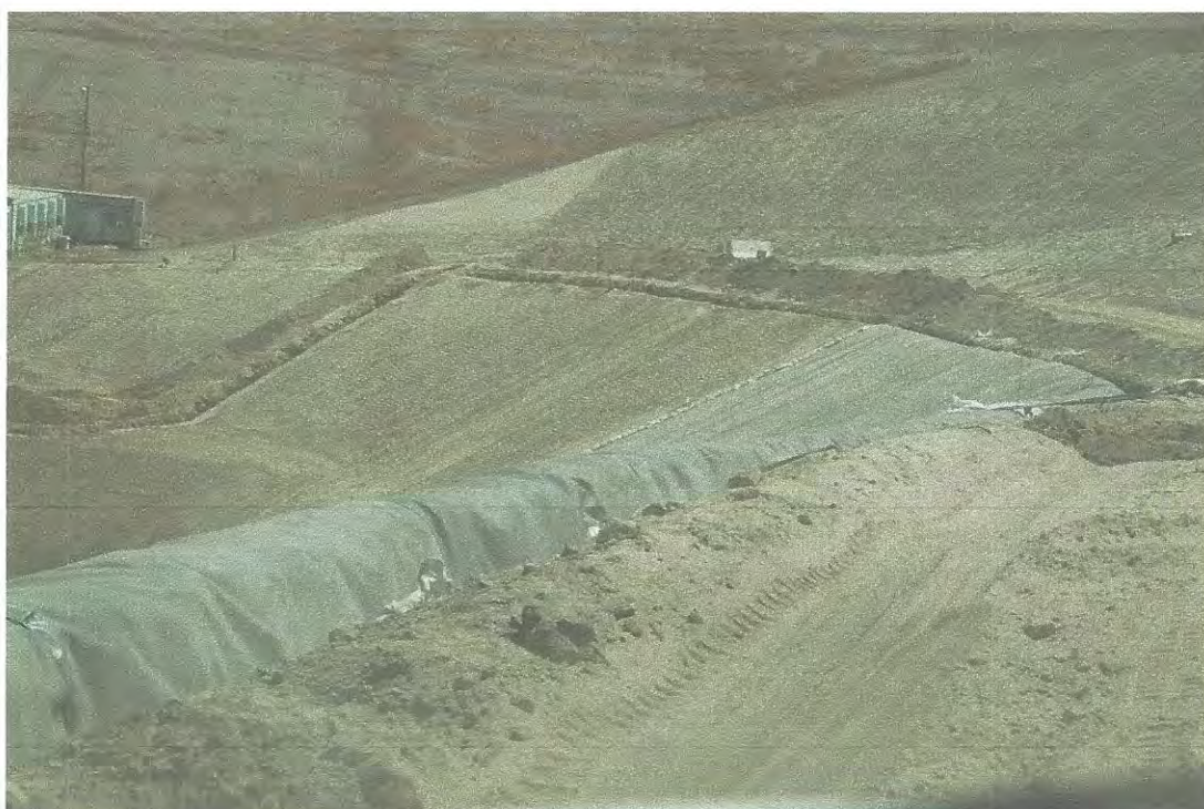
Photo 20: Anchor trench at bench of Cell CC4
