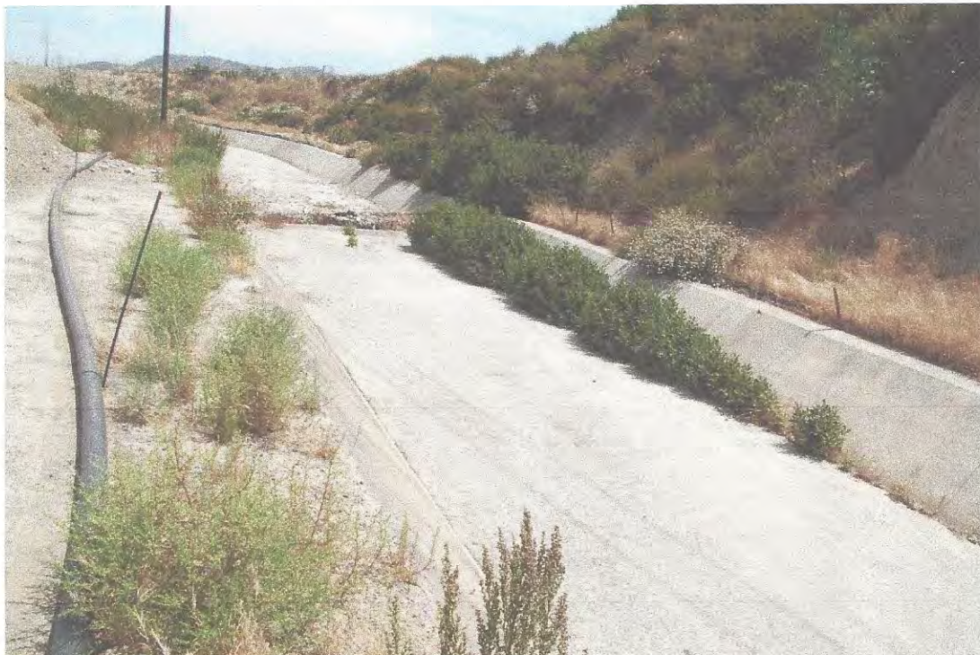
Photo 4: Vegetation growing between floor slab and wall of east perimeter channel
