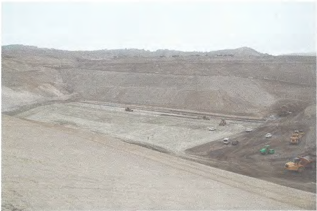
Photo 14: Placement of lower clay layer of double composite liner system
