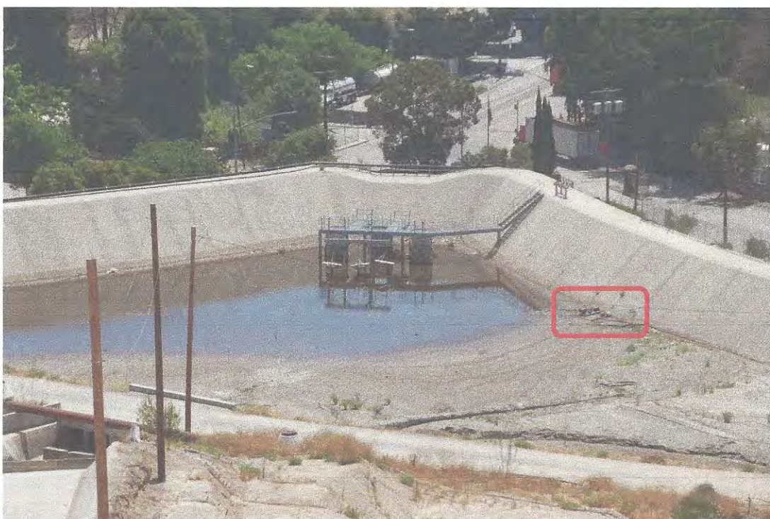
Photo 2: Terminal basin – notice pump on right side near water edge in red box
