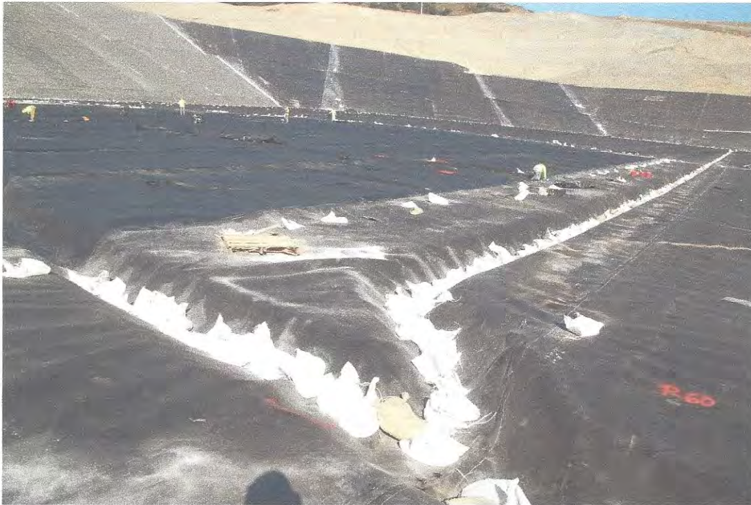
Photo 17: Sand bags in trenches for leachate collection piping at Cell CC4 Phase 4
