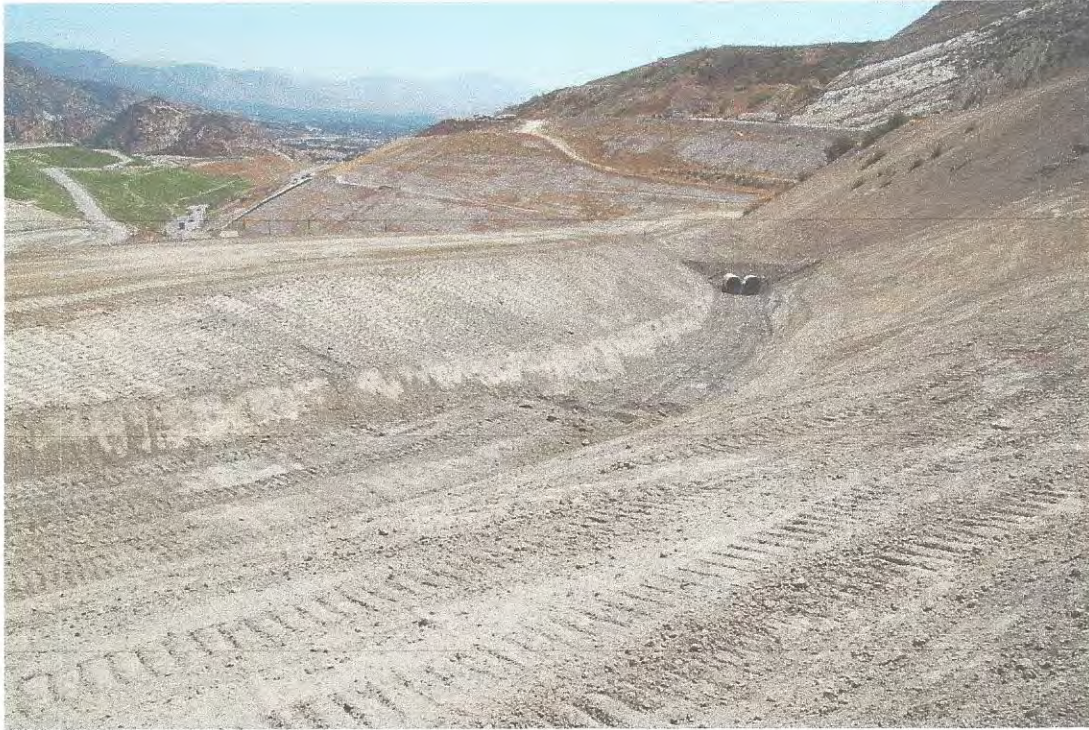
Photo 13: Detail of New Perimeter Channel on south side and perimeter road
