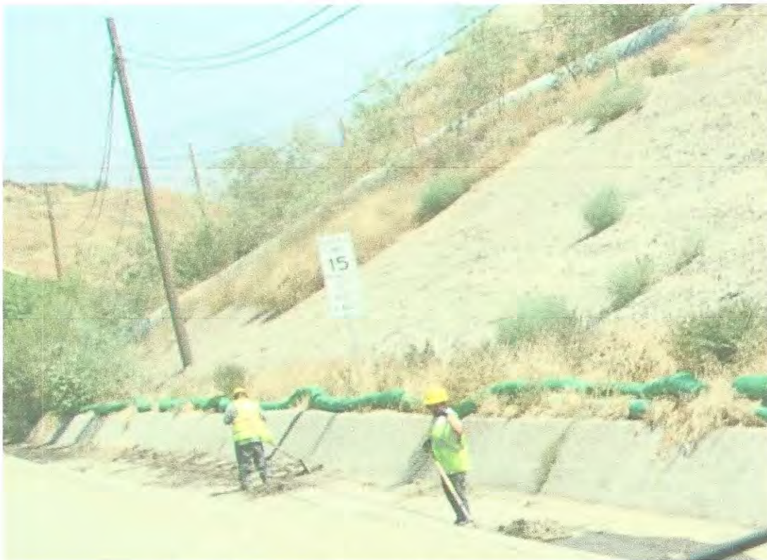
Photo 14: Clearing of channel along main access road
