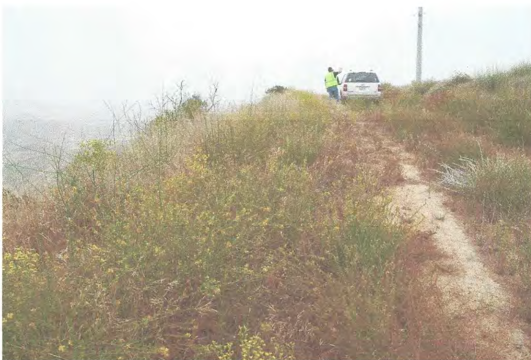
Photo 16: Ridge on south edge of landfill – no fissures or cracks noticed
