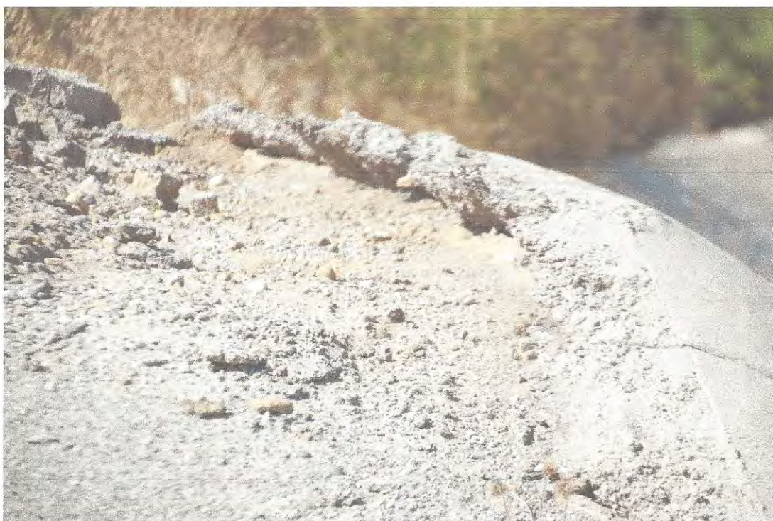
Photo 6: Undermined concrete of spillway of southern half of Basin D
