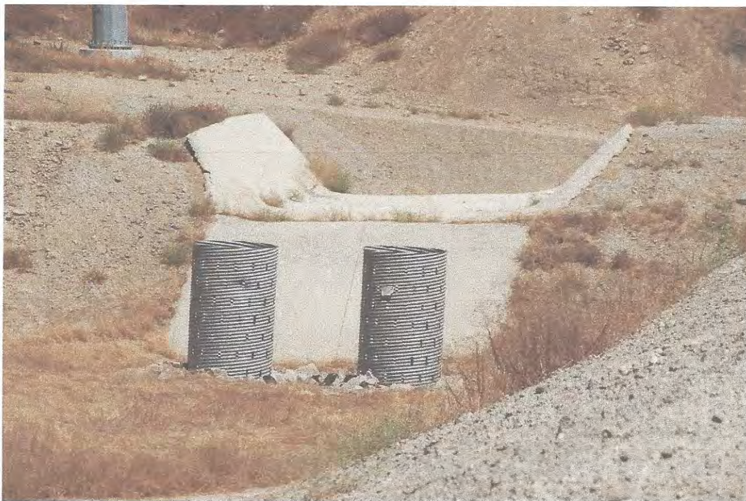
Photo 10: Missing safety guard bars on top of decant towers at northern half of Basin D
