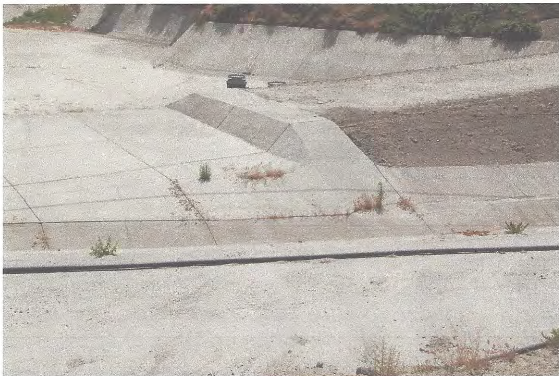
Photo 5: Vegetation in cracks in downstream side of concrete spillway at Basin B
