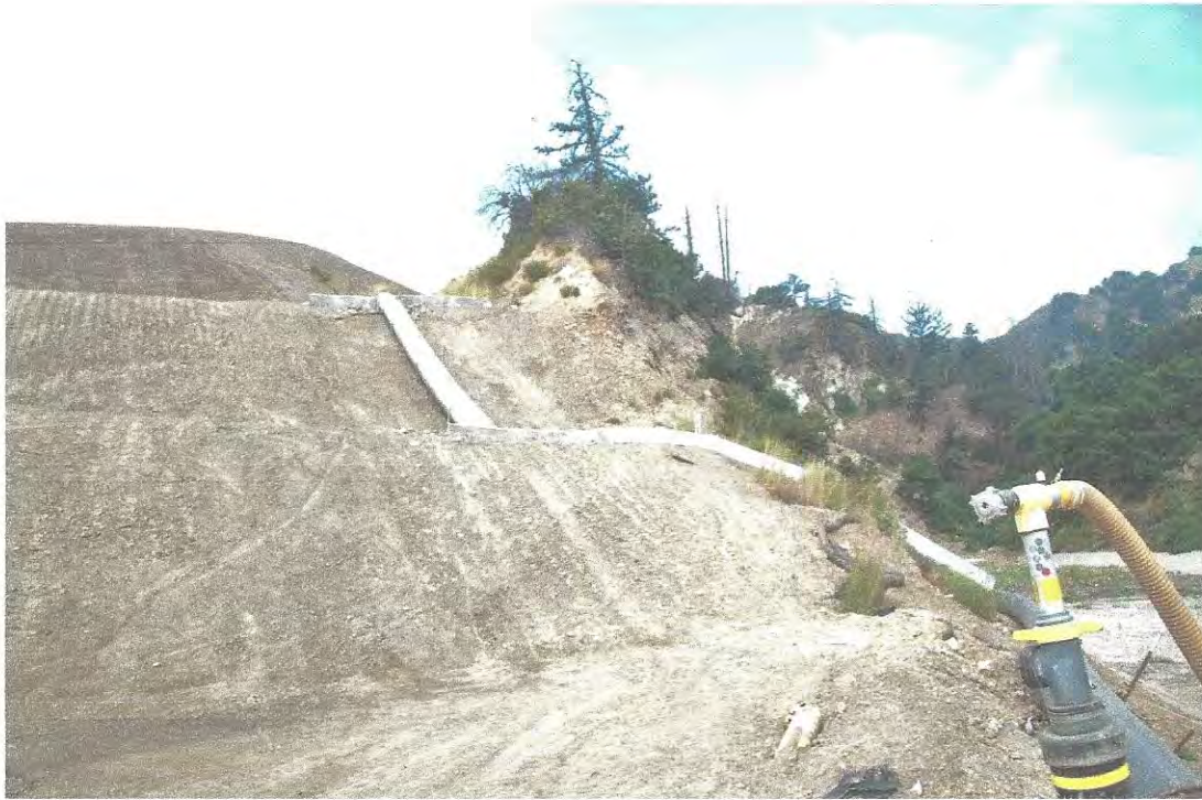
Photo 11: CMP down chute at contact between grade slope below Flare 3 and Basin A
