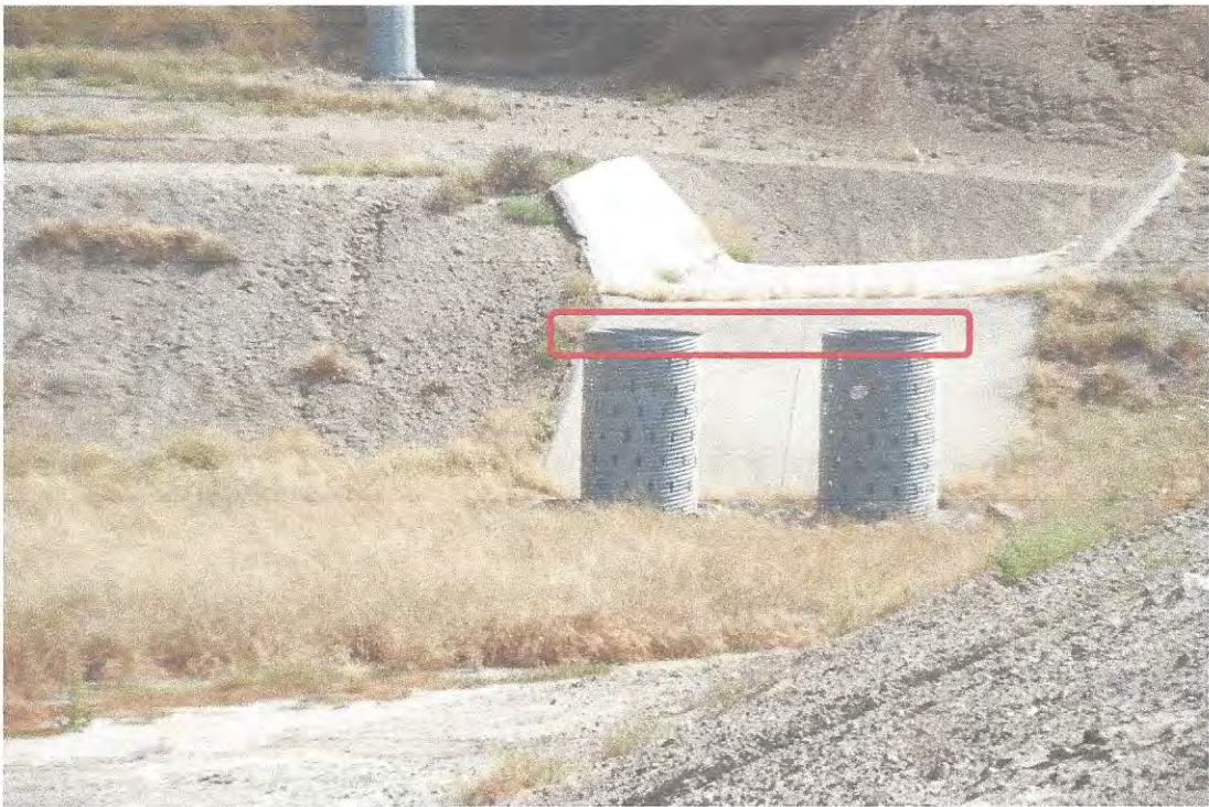
Photo 8: Missing safety guard bars on top of decant towers at northern half of Basin D
