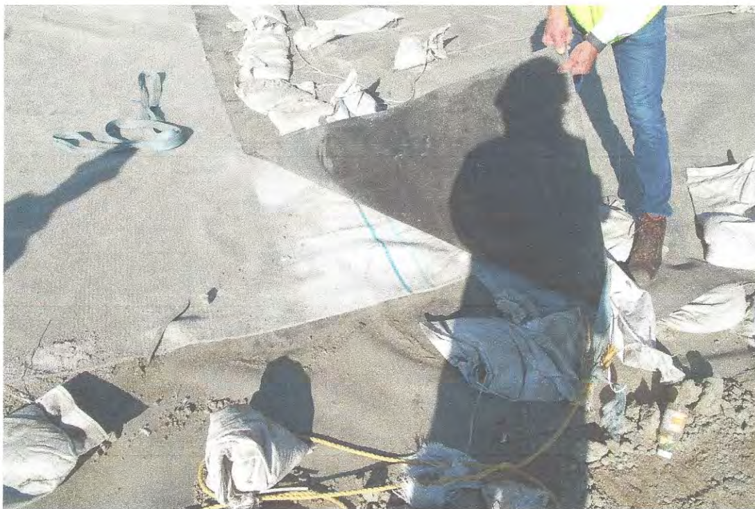
Photo 19: Liner system on slopes of Cell CC4 Phase including GCL
