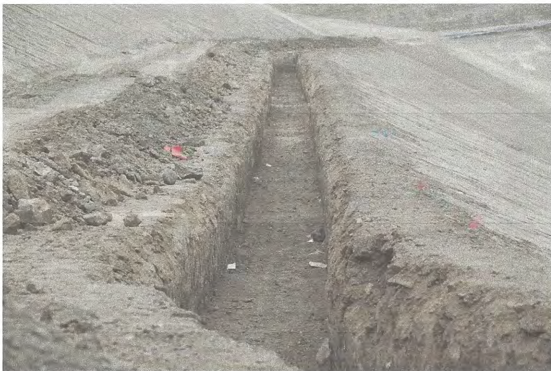
Photo 15: Anchor trench for geosynthetics at Cell CC4 Phase 4
