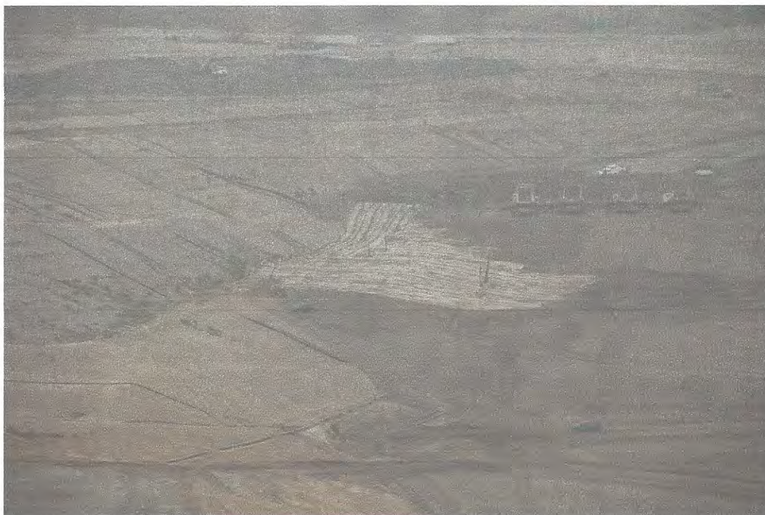
Photo 1: Daily alternative cover and tippers at waste face on cell CC4
