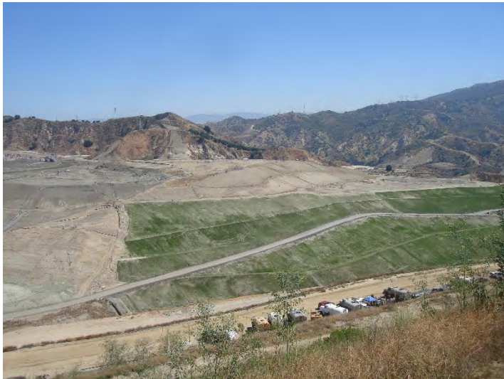
Photo 187: Closure Turf: August 13, 2019
