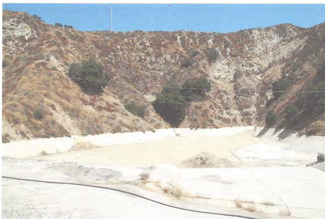
Photo 8: Sediment accumulation in Basin B
