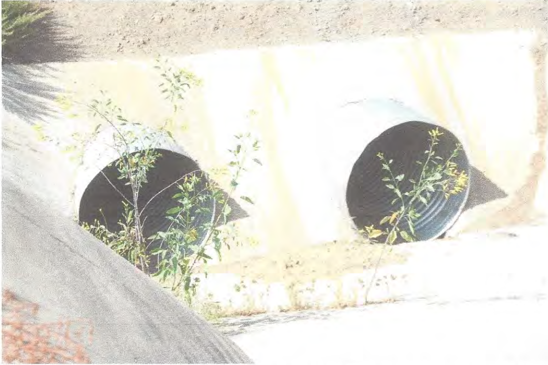
Photo 7: Vegetation growing in downstream side of concrete of spillway of southern half of Basin D
