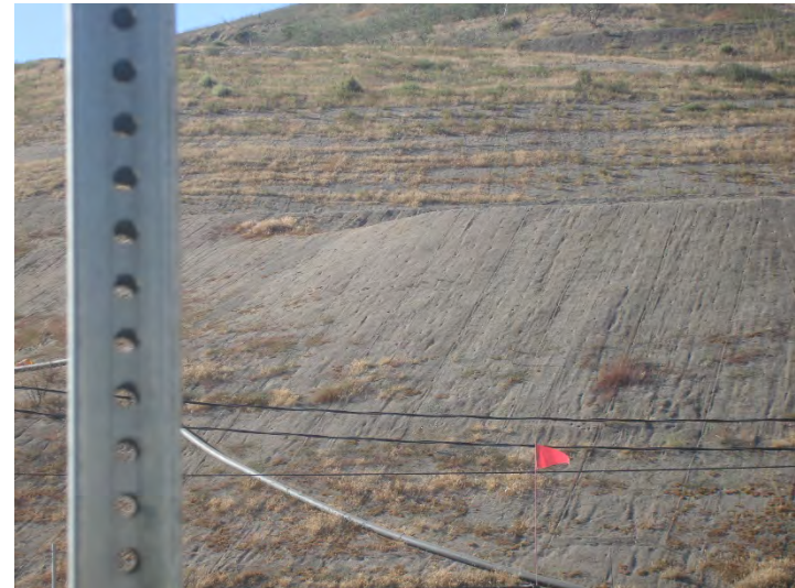
Photo 244: Old City South Stockpiled Soil Slump: August 13, 2019
