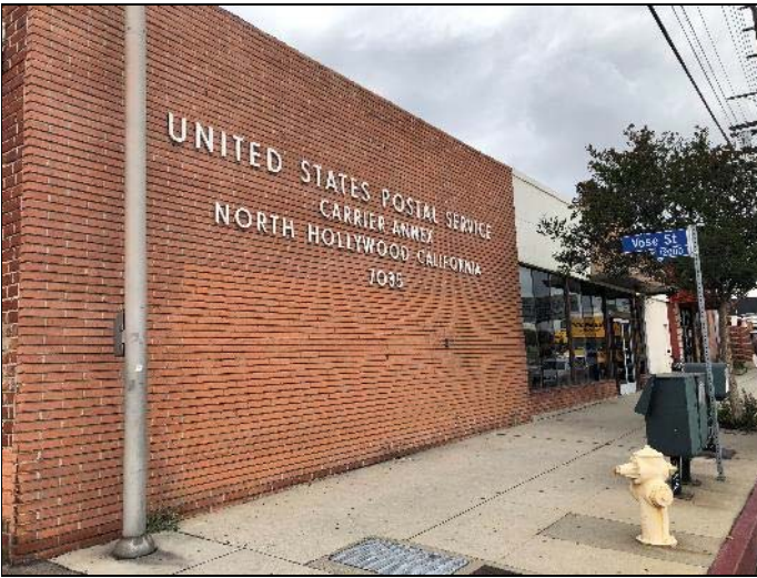
1. View of subject property east elevation.
