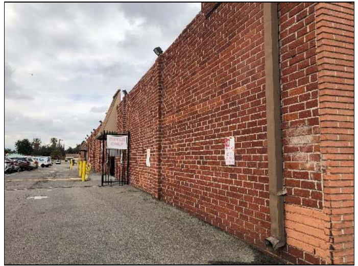
2. View of south elevation.
