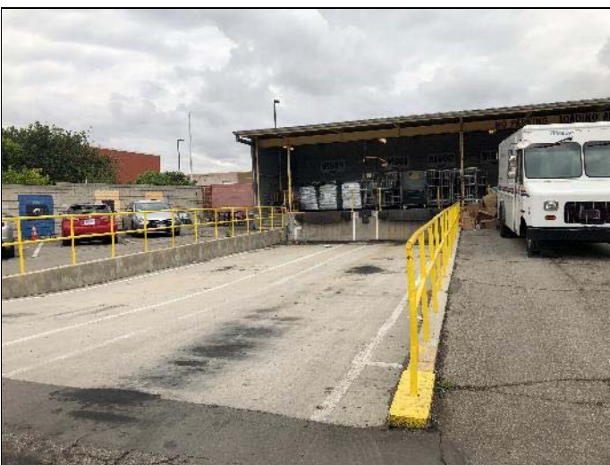
17. View of loading dock.
