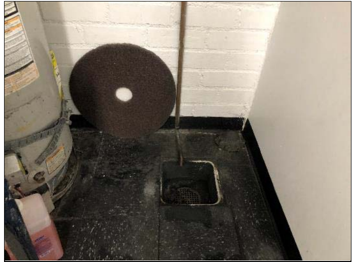
14. View of floor drain in storage room.
