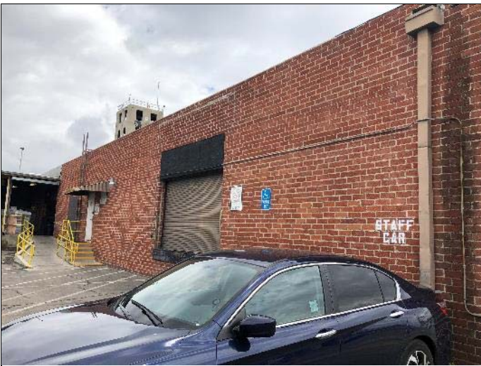
3. View of west elevation.
