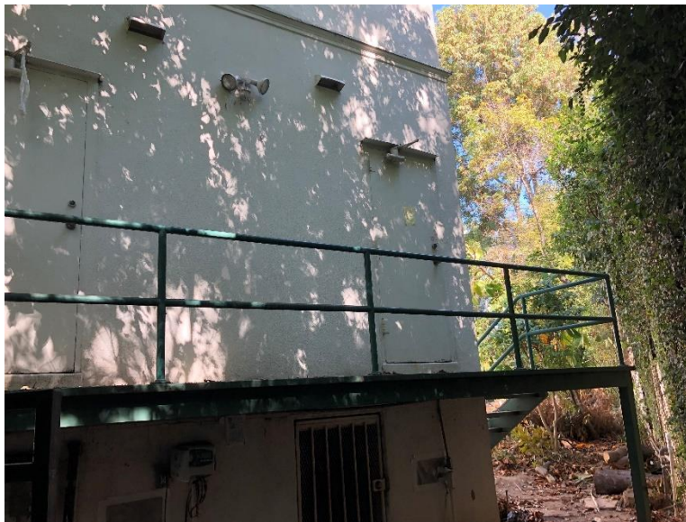
Figure 16. Southern Façade SOURCE: Sapphos Environmental, Inc., 2019
