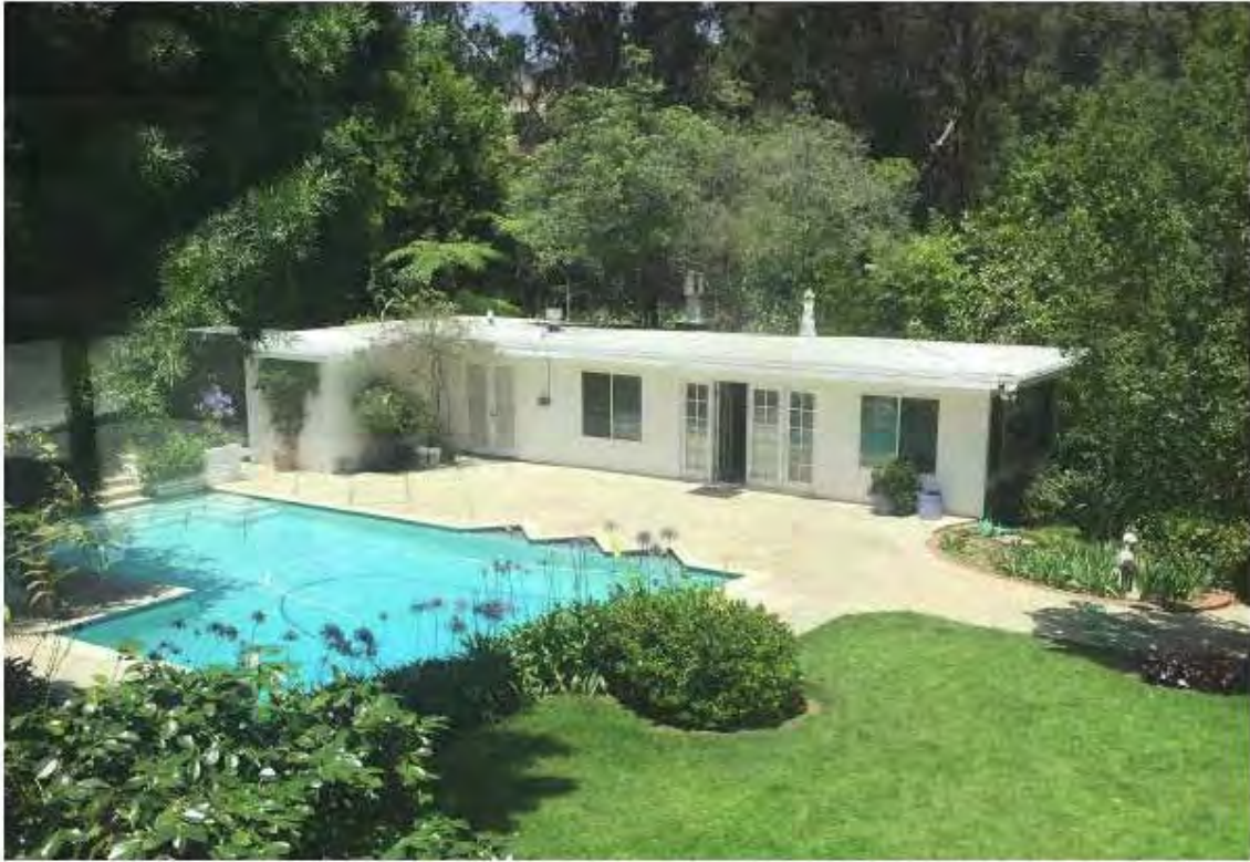
Weinberg Residence, pool and pool house, 100 Delfern Drive, July 2019, (Ron Woodson photo)
