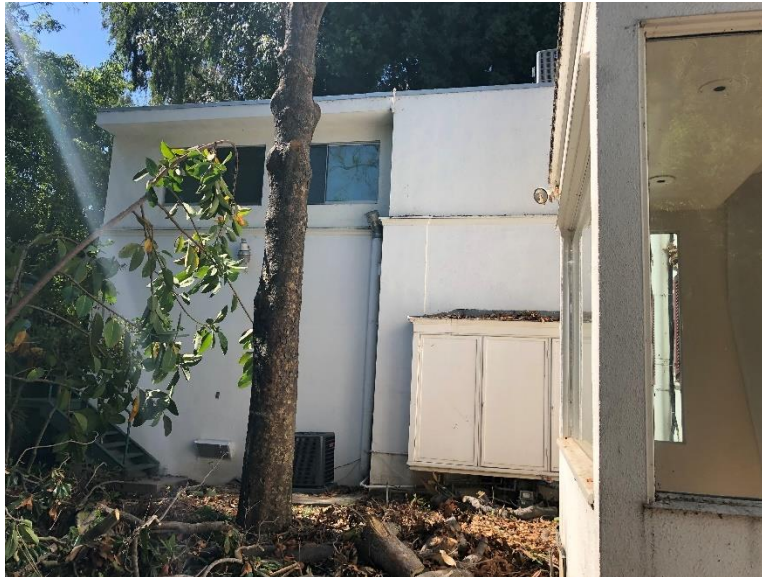
Southern End of Eastern Façade
