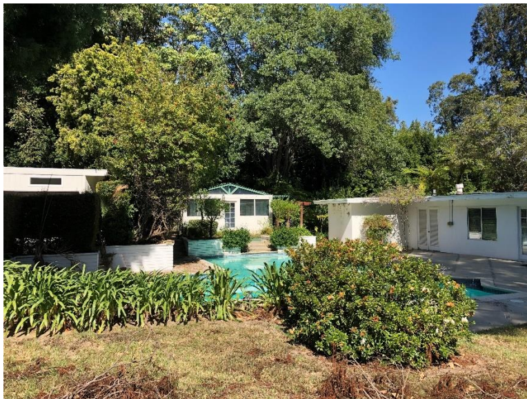
Garage Addition (left of frame)
