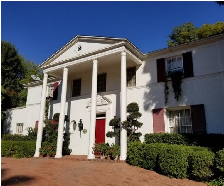
View of Primary (Western) Façade
