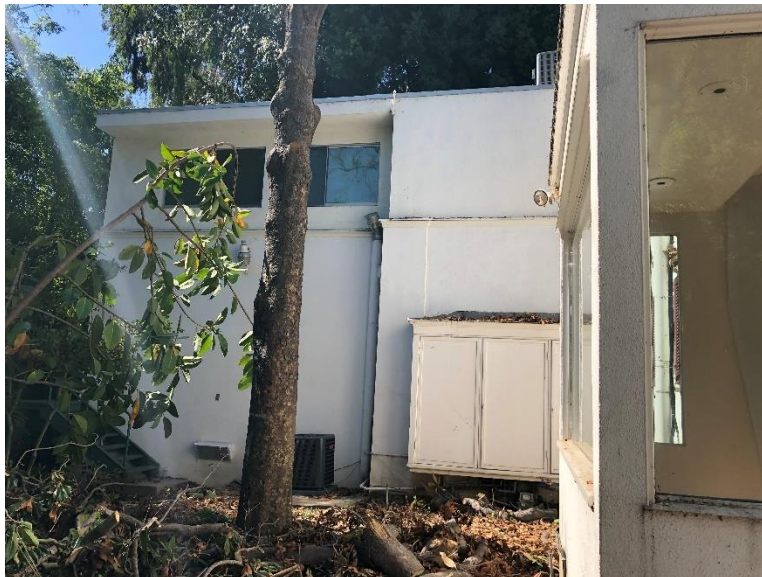
Figure 14. Southern End of Eastern Façade
