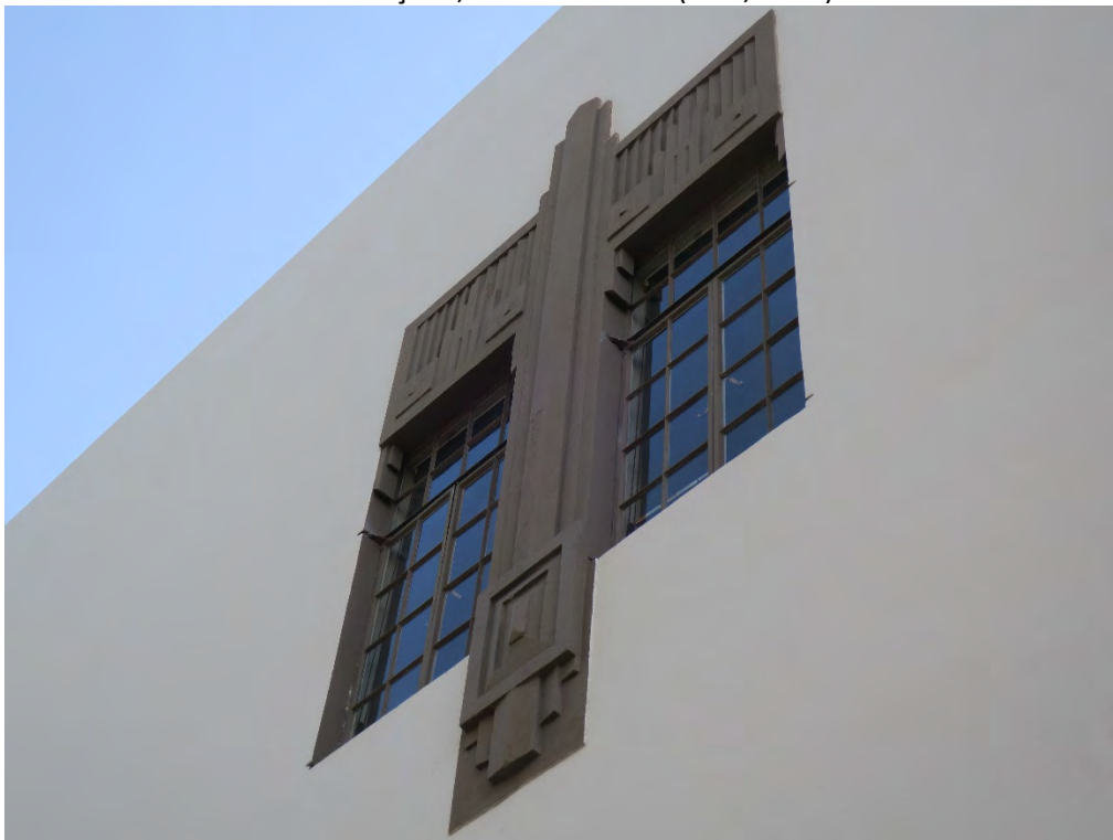
Art Deco details at north (primary) façade (ARG, 2019).
