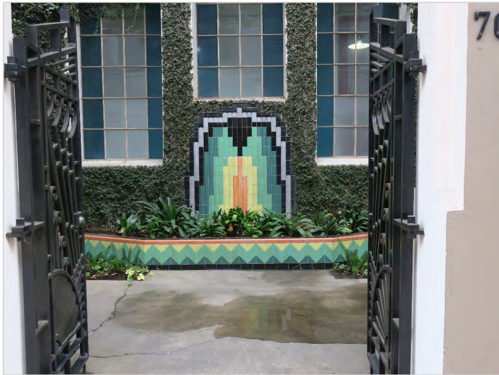
Detail of entry gates and tiled planter, view south (ARG, 2017).
