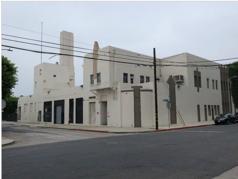
East façade and portion of north façade, view southwest (ARG, 2017).
