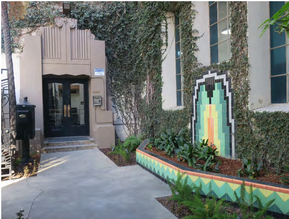
Primary entrance and tile planter, view southeast (ARG, 2019).
