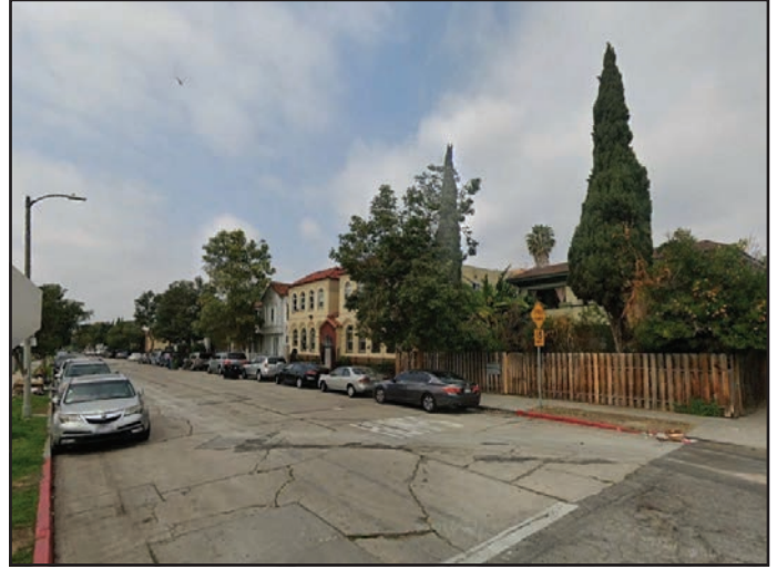
View 2: View to the northwest of the one- and two-story residential uses.
