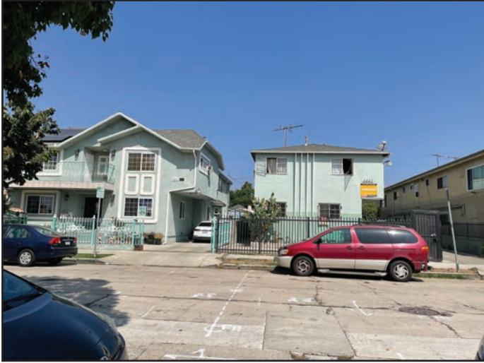
View 1: View to the north of the two-story residential uses.
