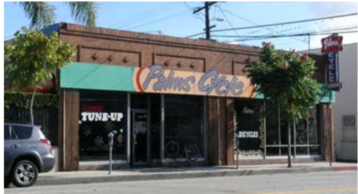
3770 S. Motor Avenue, 1923 Long-time home of Palms Cycle Shop; Palms Cycle was established here in 1930. (SurveyLA)
