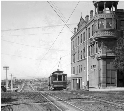
View looking west on 1st Street at Boyle Avenue (ca. 1895), California State Library Image Archive
