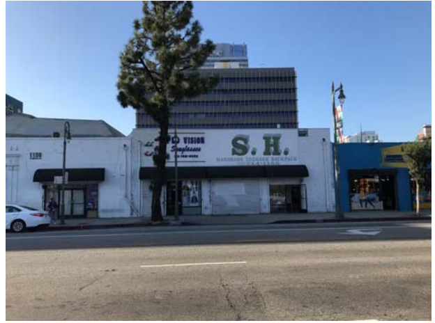
20. View of south adjacent
