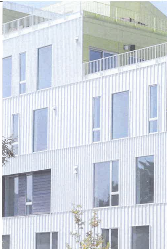
EXTERIOR FACADE MATERIAL - VARIATION IN CORRUGATED METAL CLADDING
