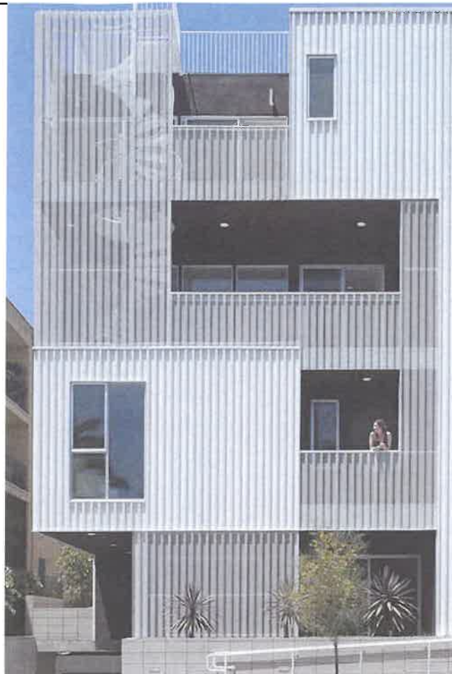
EXTERIOR FACADE - TRANSPARENCY THRU PERFORATION OF METAL CLADDING
