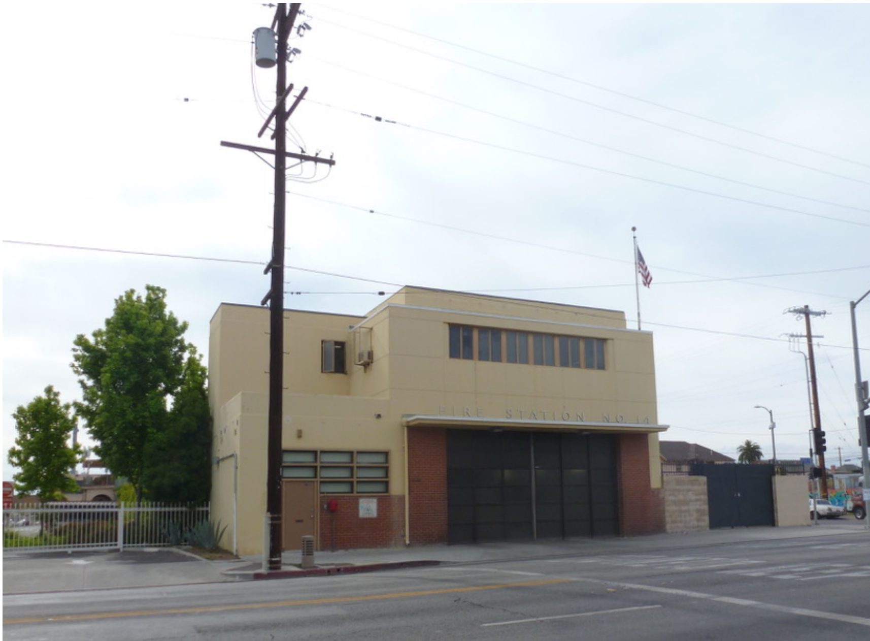
Fire Station No. 14, view of east elevation, looking west (Teresa Grimes, April 2021)
