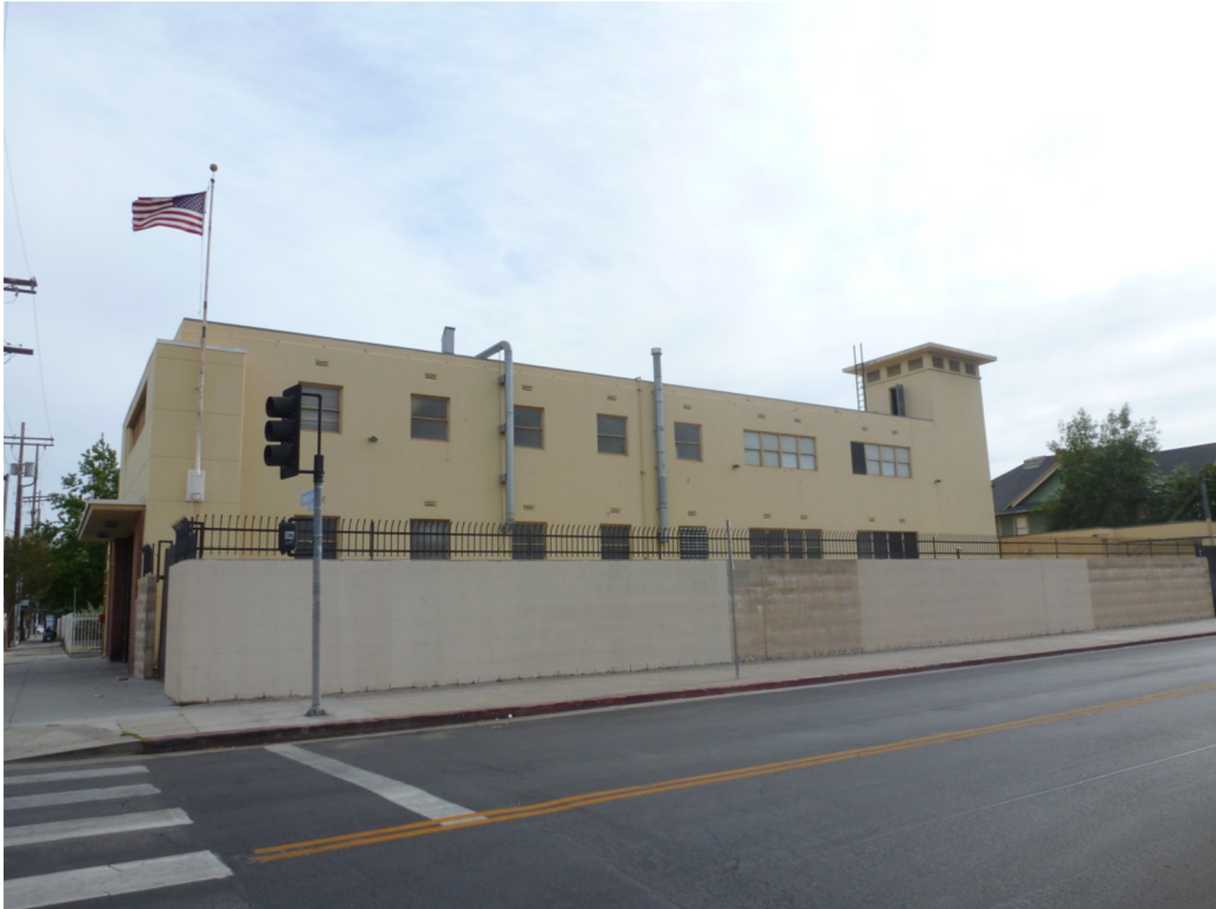
Fire Station No. 14, view of north elevation, looking south (Teresa Grimes, April 2021)
