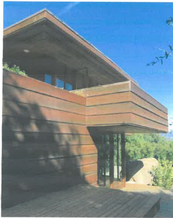
View northeast of the second story balcony at the south façade (ARG, 2019).
