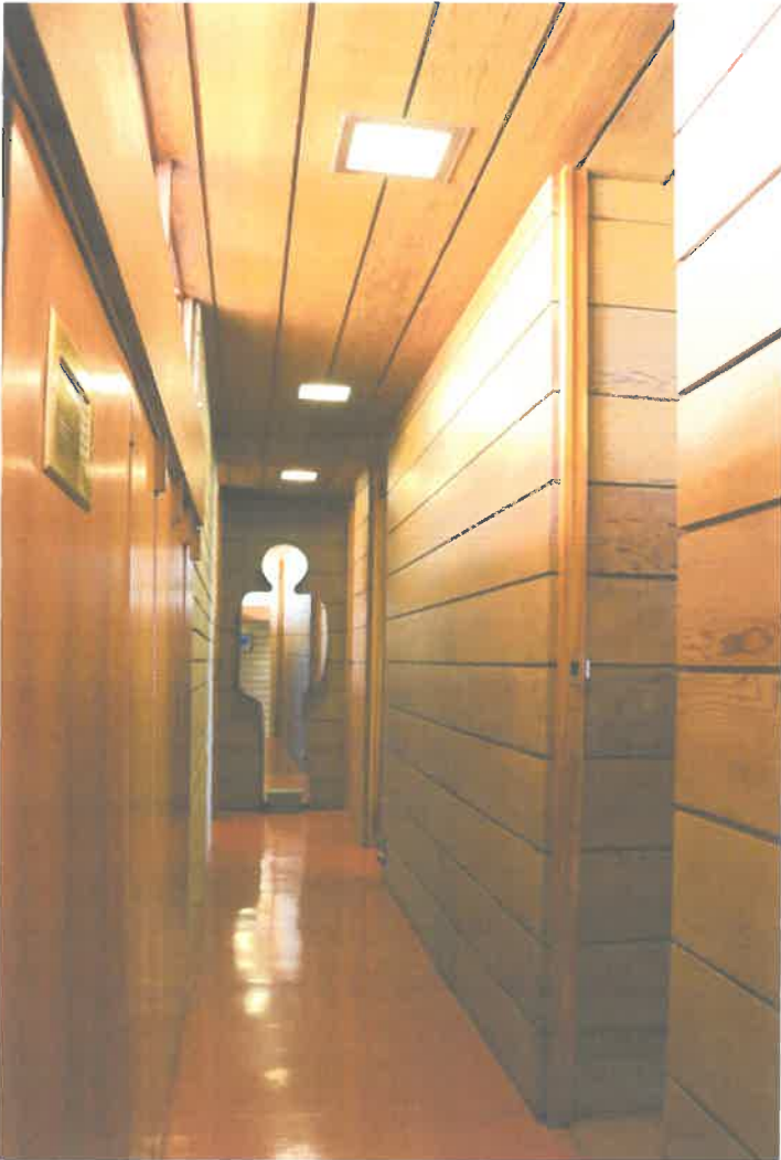
Redwood channel paneling in main hallway looking toward bedrooms.
