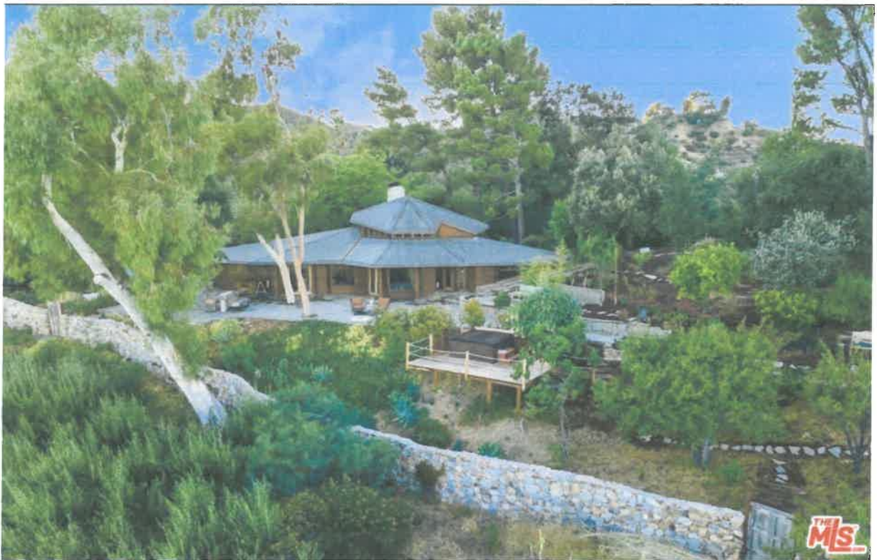
1963 Wear Residence, 2440 Minard Road, Topanga Canyon
