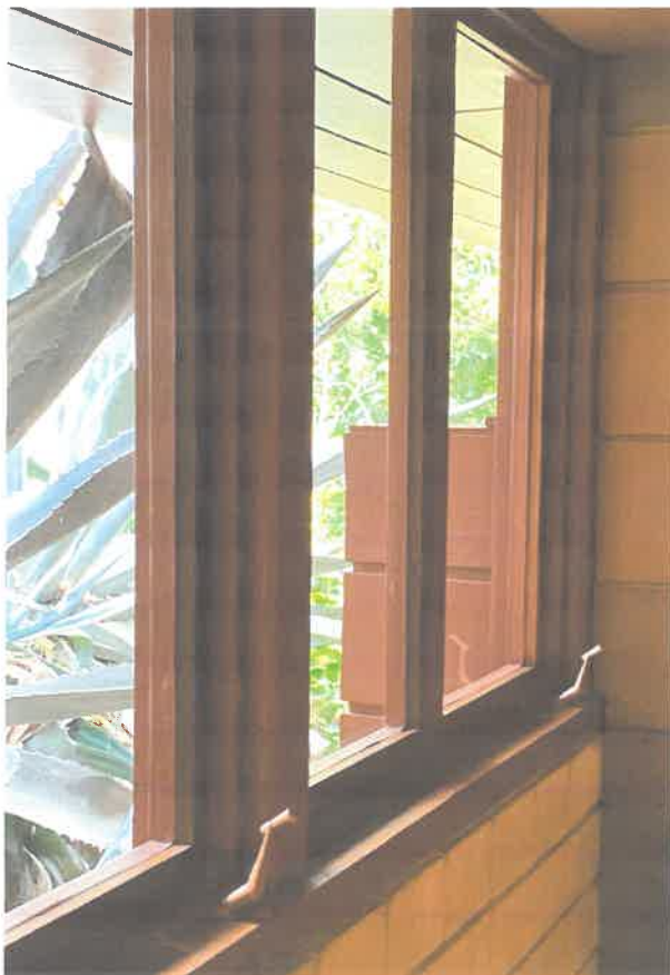
Above - Study looking north with high fixed units and tall casement windows facing the view.
