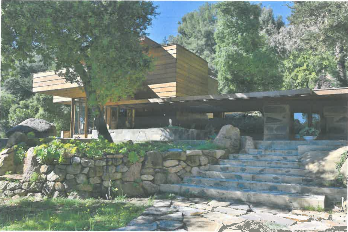
1958 Anderson House. 19974 Sischo Drive, Topanga Canyon Listed as a Los Angeles County Landmark in 2019 (nomination attached)
