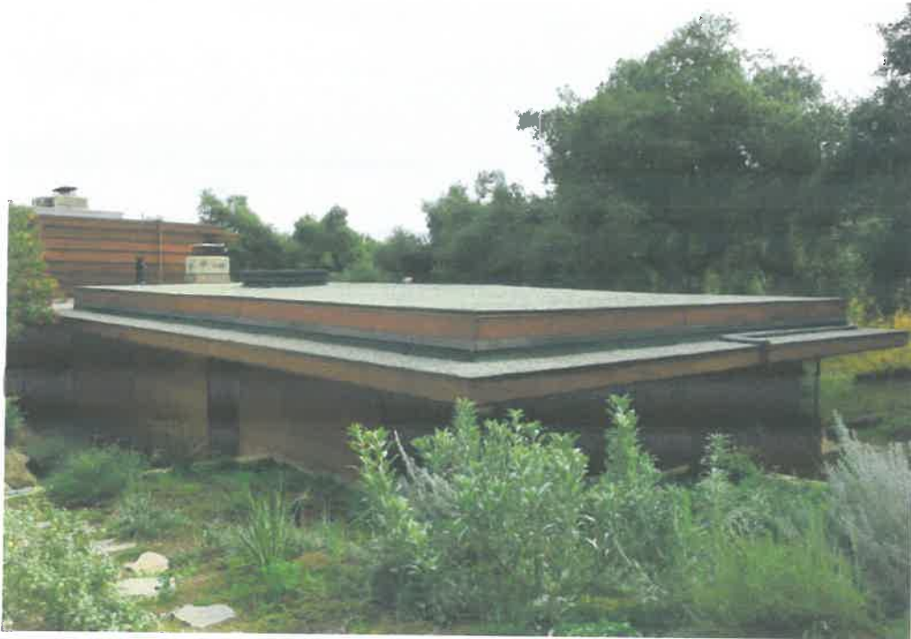
View southeast of the north and west façades (ARG, 2019).
