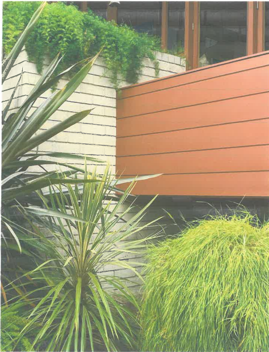
Detail of retaining wall at exterior deck with planter on top.
