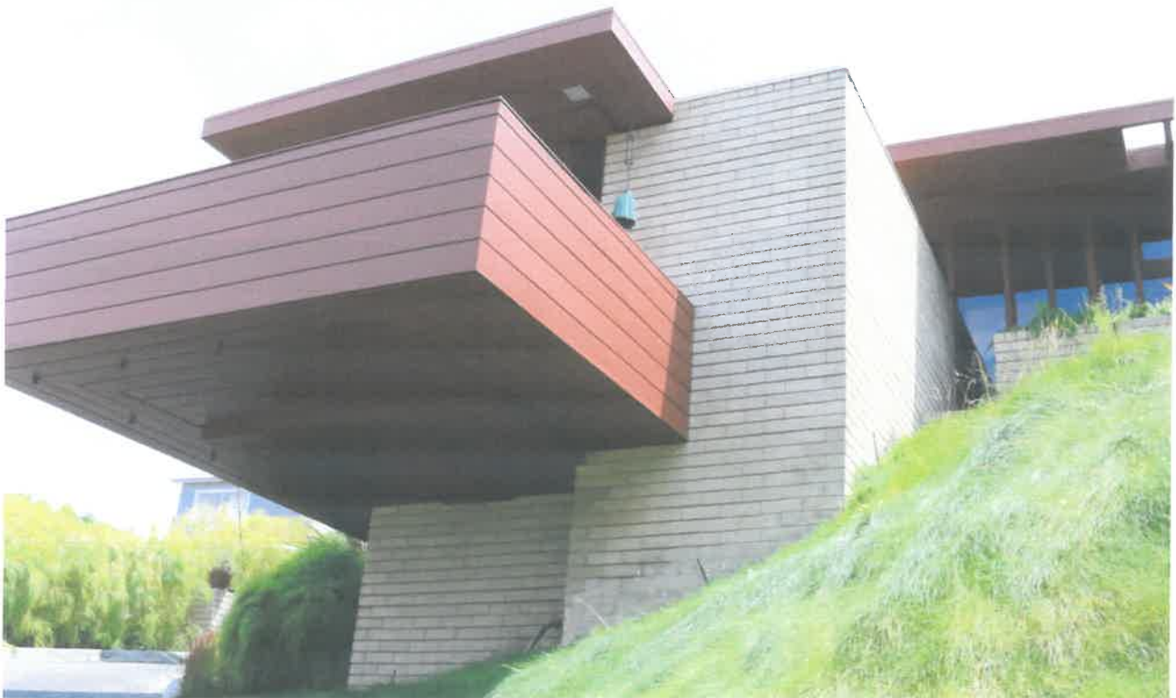
View looking south near the top of the driveway.
