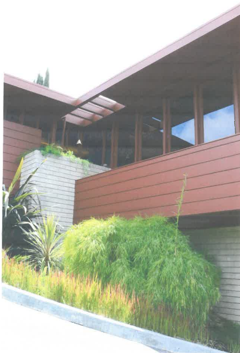
View looking southwest with trellis over original masonry planter.
