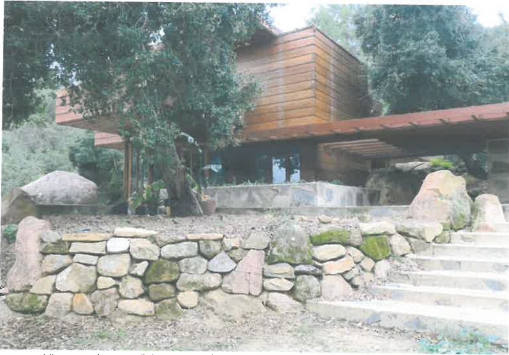
View southwest of the carport/entrance canopy and east façade (ARG, 2019).
