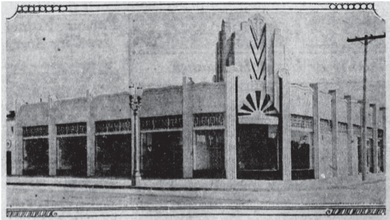
"Modernistic Type Store Building," Los Angeles Times , May 3, 1931.
