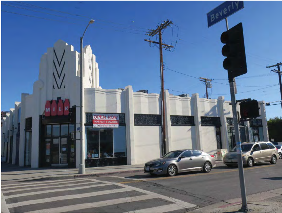
West façade, view east (ARG, 2021).
