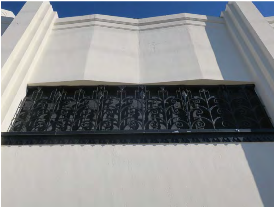
Detail: zig zag parapet and wrought iron grille (ARG, 2021).
