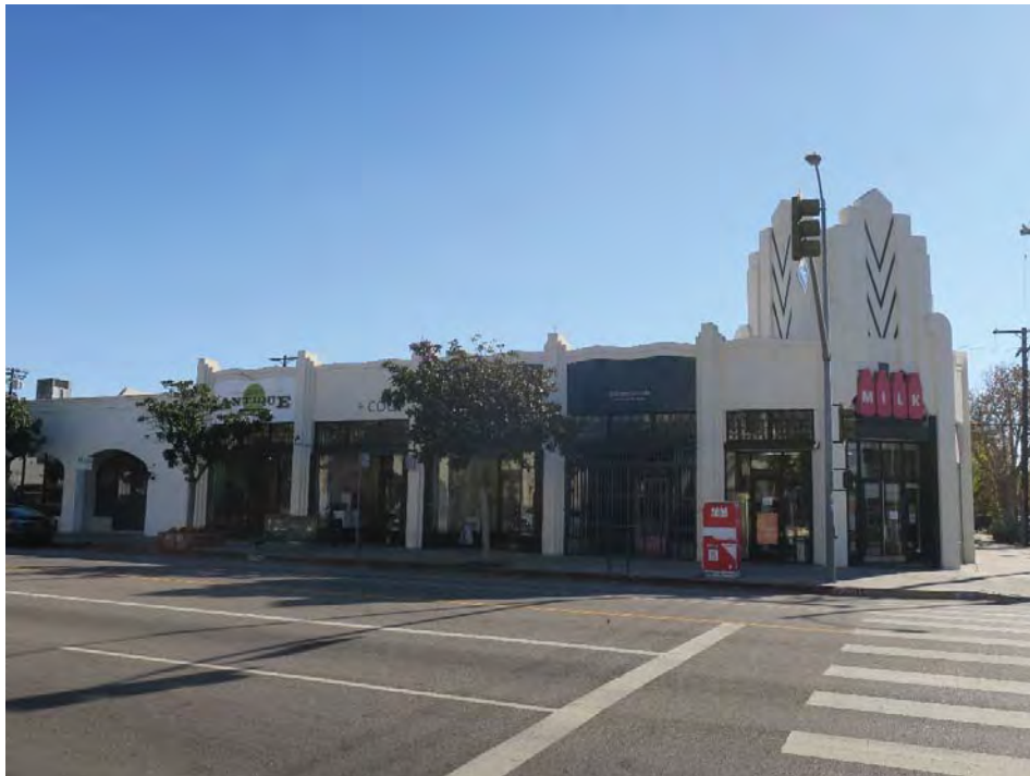
Primary (north) façade, view south (ARG, 2021).
