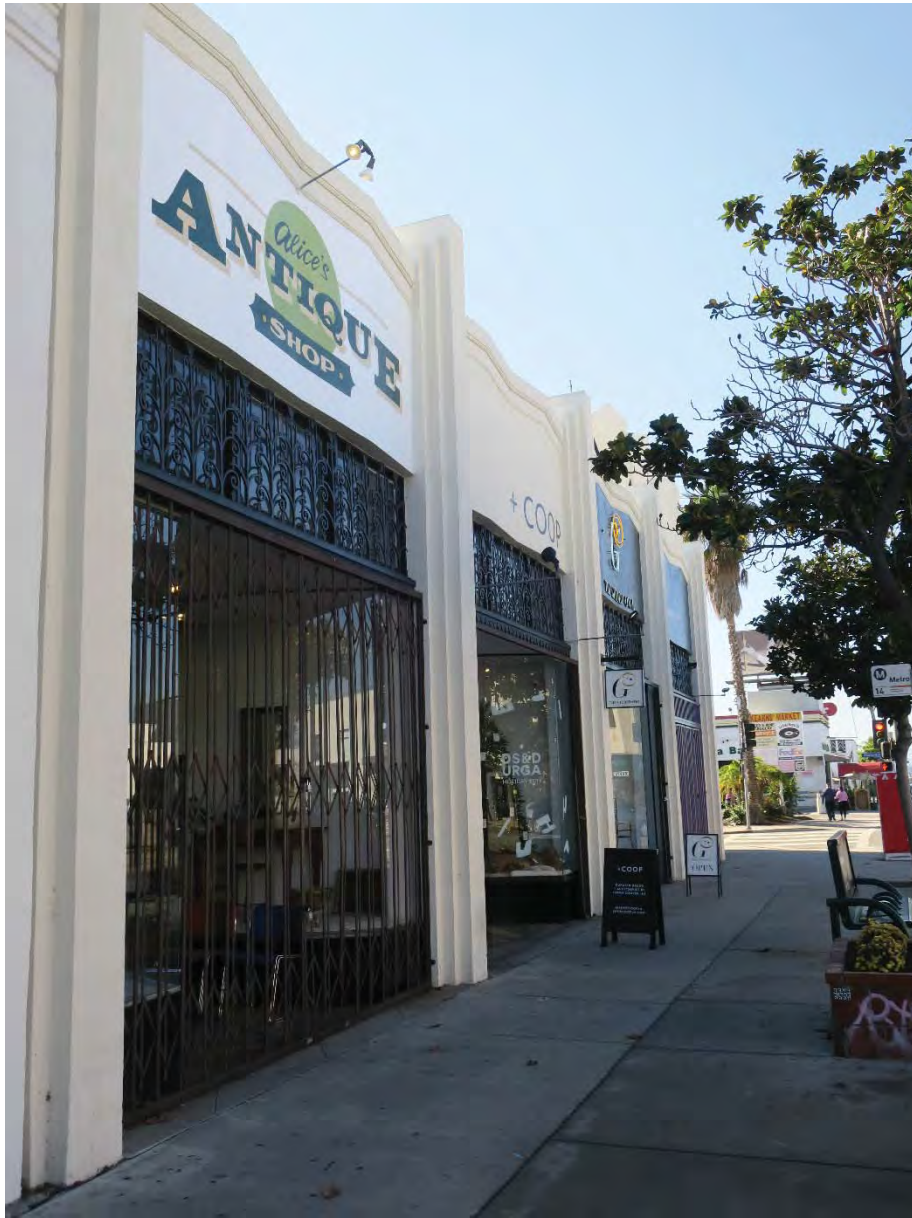
North façade, view west (ARG, 2021).
