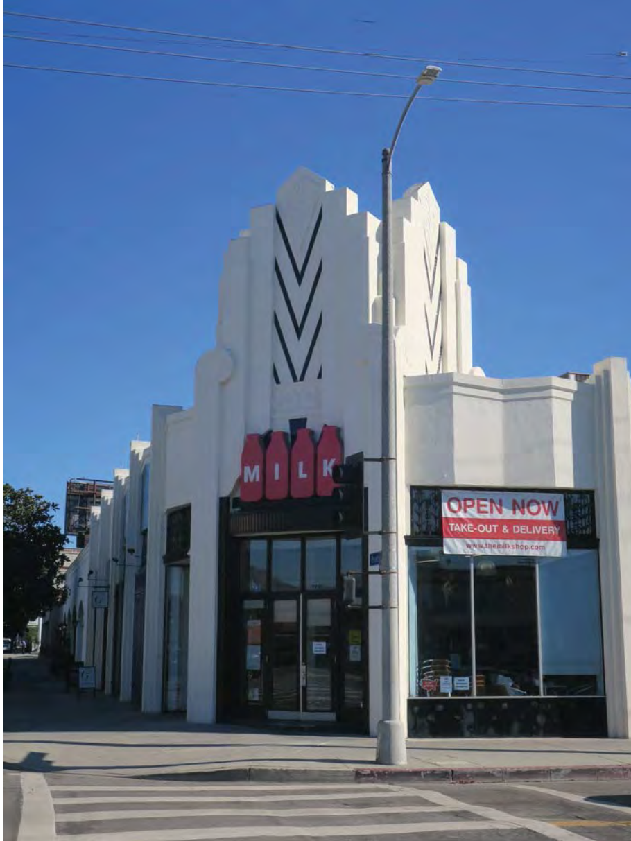
Northwest corner façade, view east (ARG, 2021).
