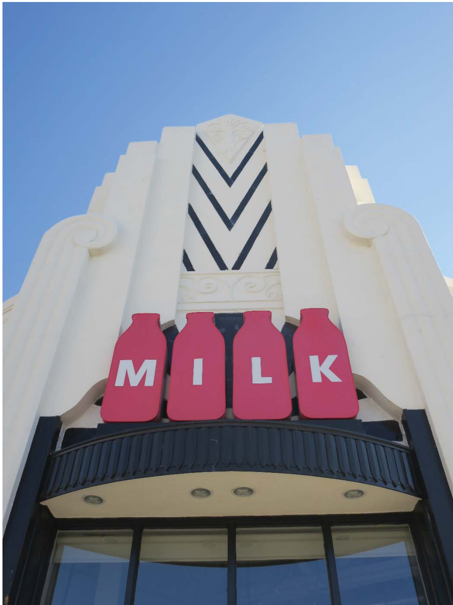
Detail: corner tower, view southeast (ARG, 2021).
