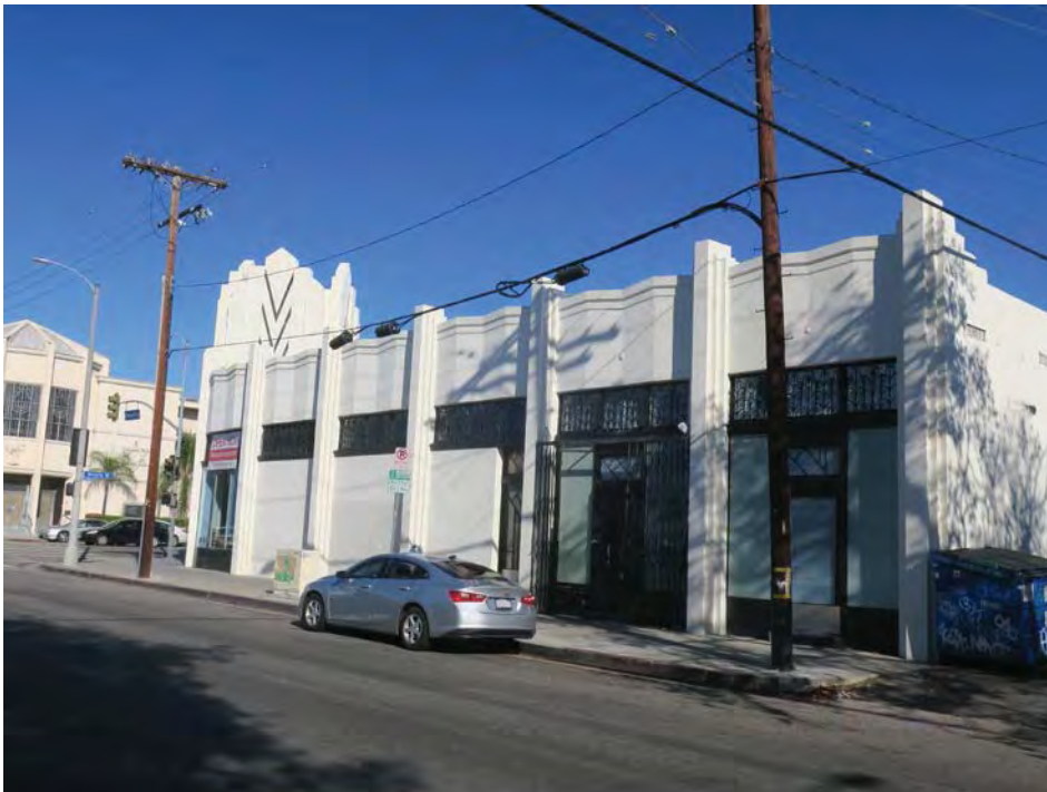
West façade, view northeast (ARG, 2021).
