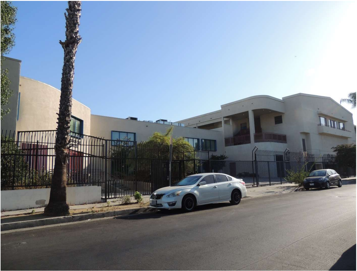
Primary (south) façade, view looking northeast.
