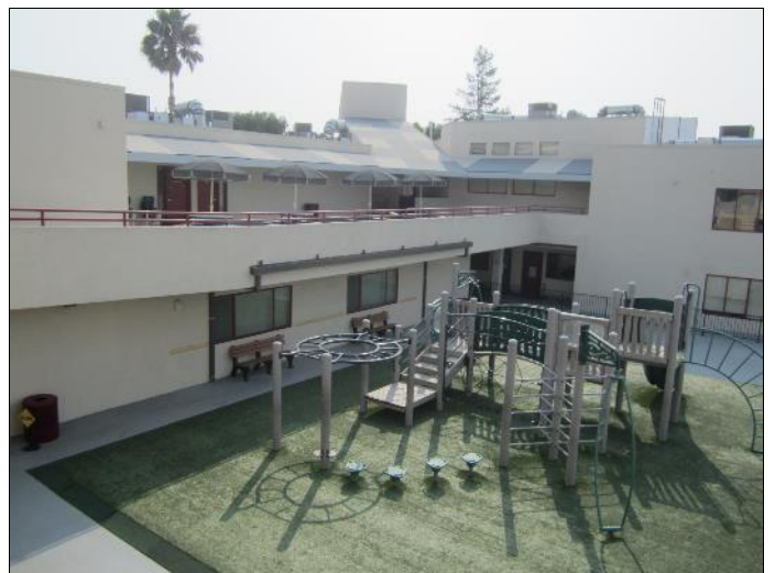
6. Northern side of the subject building.
