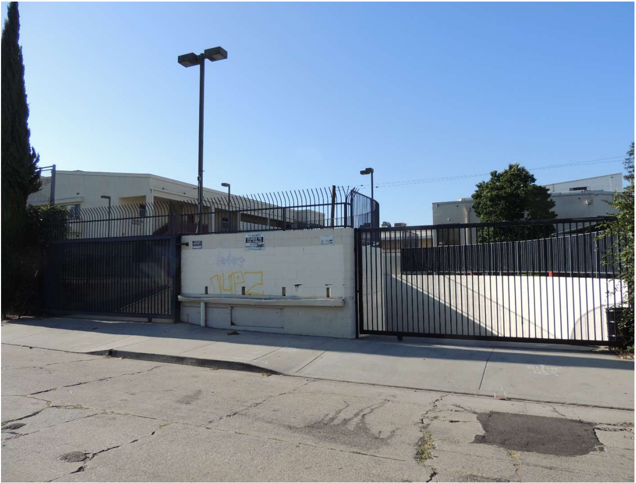
Vehicle entrance, view looking south from West La Mirada Avenue.
