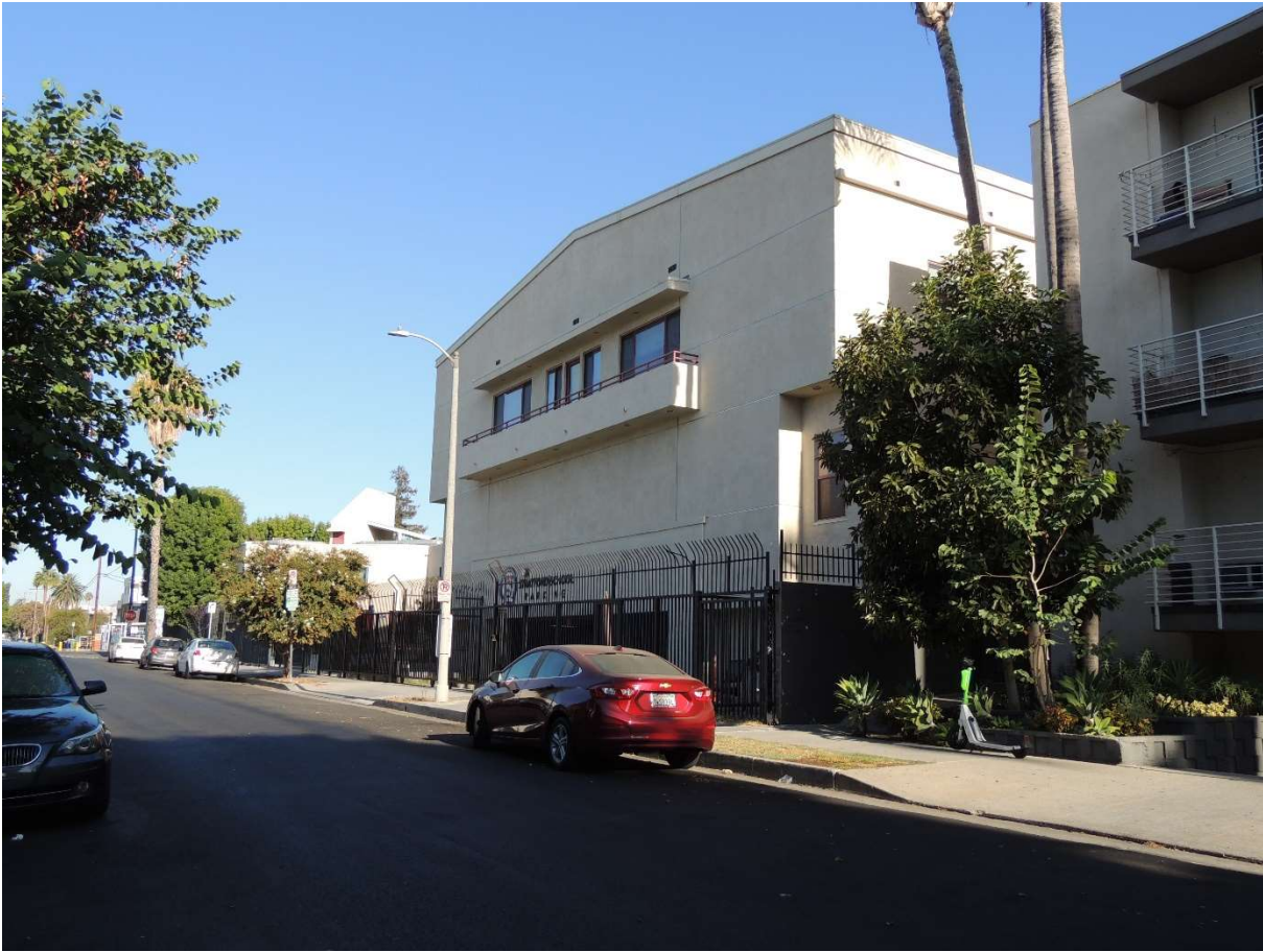
View looking northwest across West Lexington Avenue toward the subject property at 1200 North Cahuenga Boulevard.
