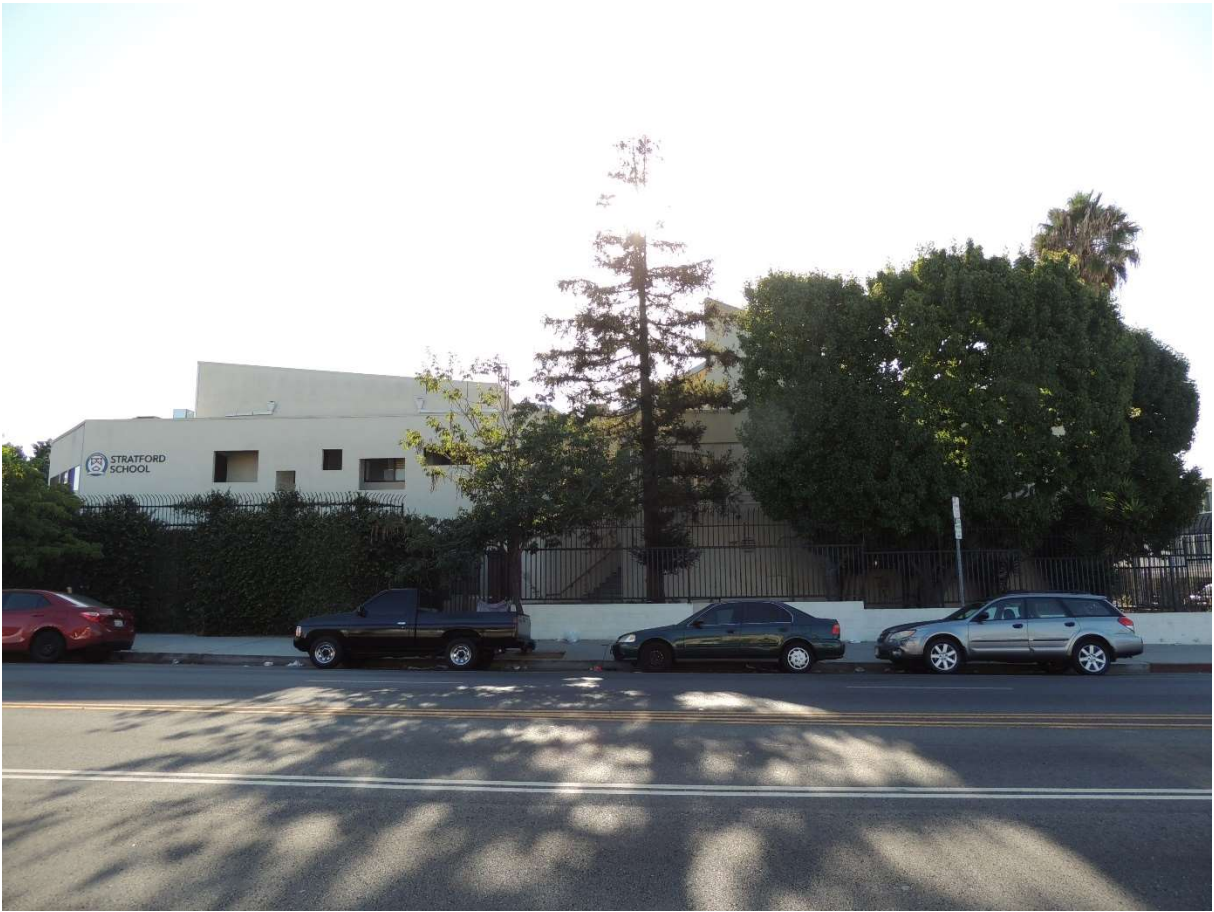
West façade, view looking east across North Cahuenga Boulevard.
