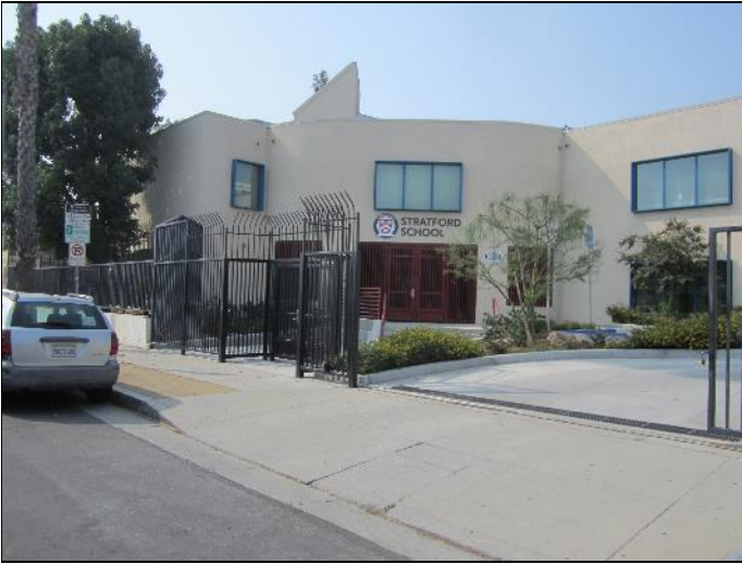
1. View of the main entrance to the subject property.
