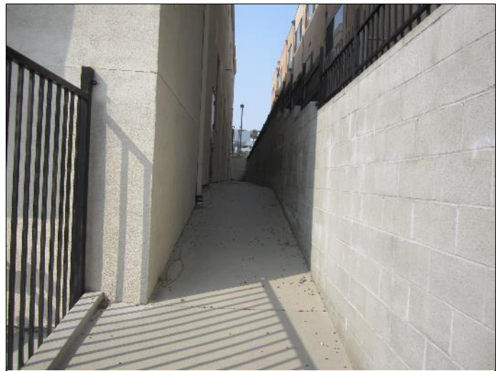
4. Eastern side of the subject property.
