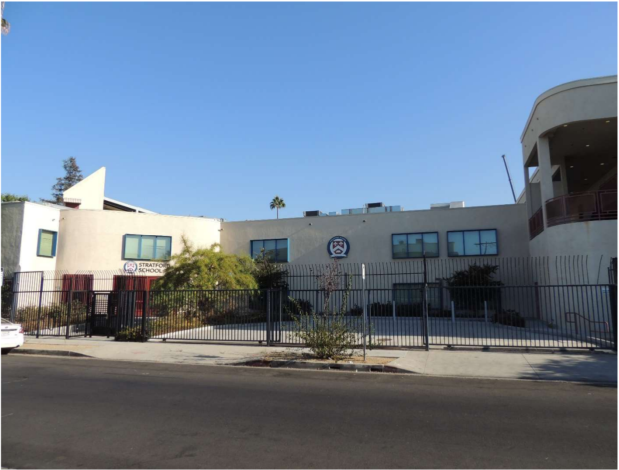
Primary (south) façade, view looking north.
