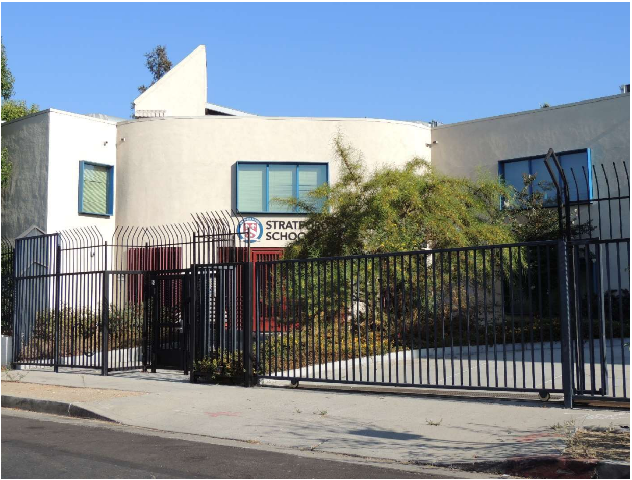
Primary entrance, primary (south) façade, view looking northwest.
