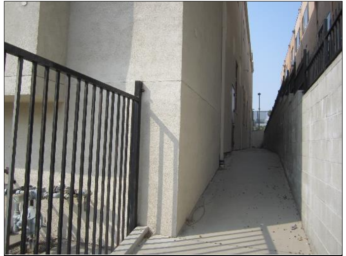
8. Eastern side of the subject building.
