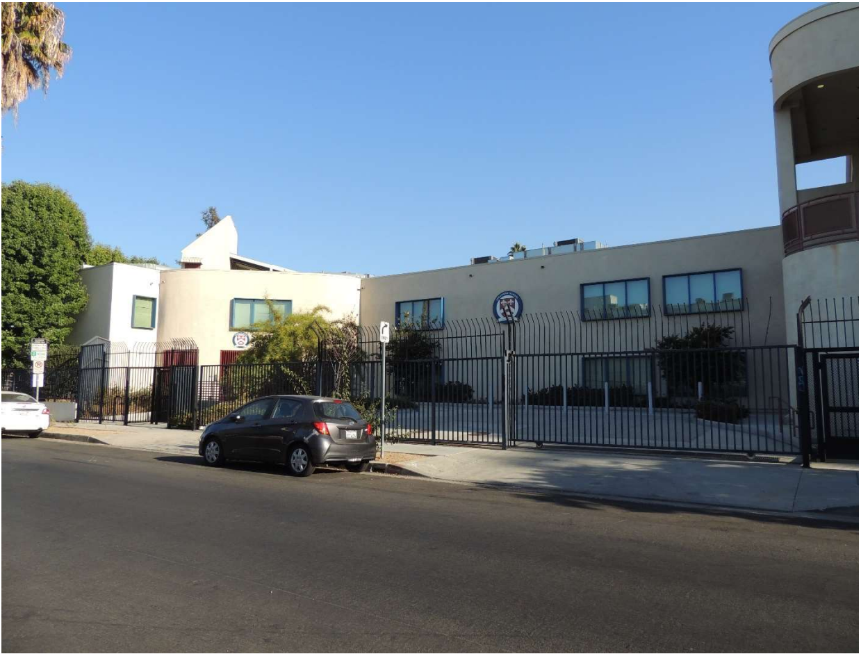
Primary (south) façade, view looking northwest.
