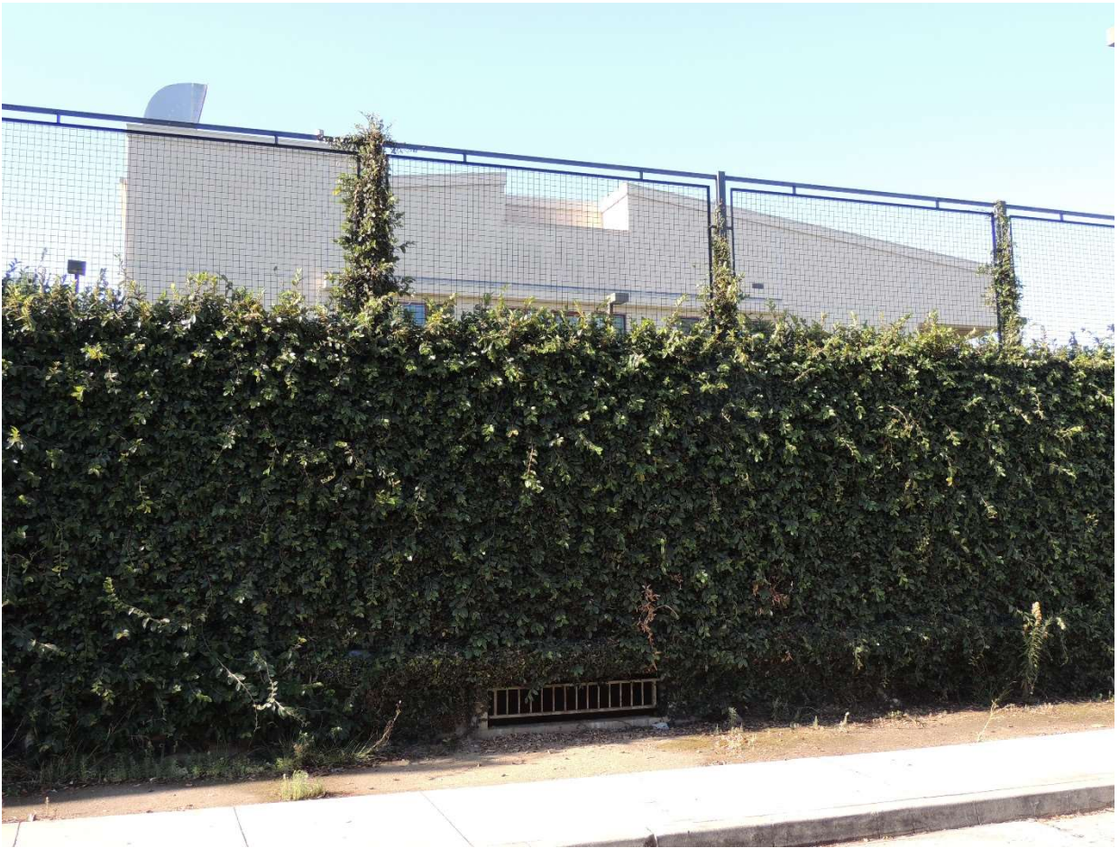
Wall detail, view looking south from West La Mirada Avenue.
