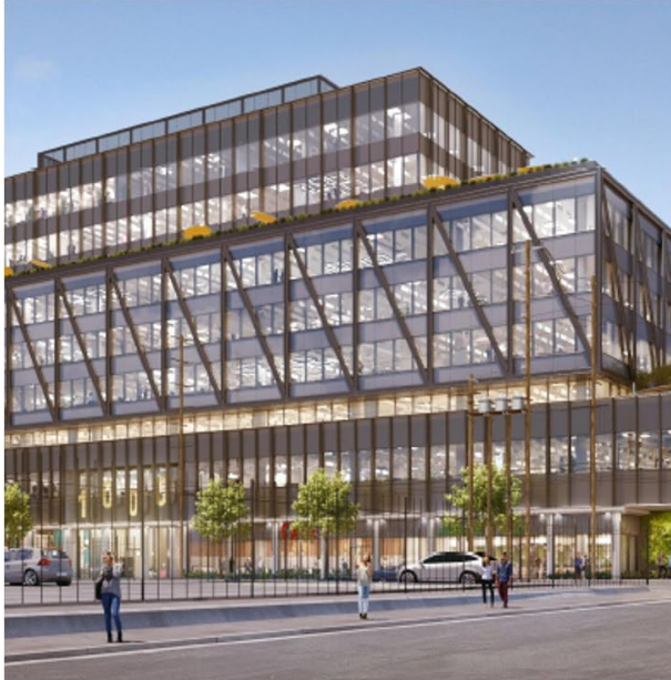
South facing Frontage (Romaine St)
