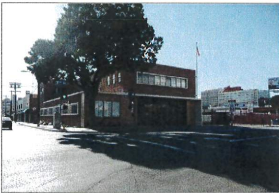
Name: Fire Station No. 9 Address: 430 E. Seventh St. Architect: Orr, Strange and Inslee Date: 1959
