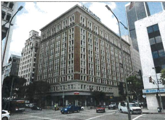
Name: Pacific Finance Building Address: 510 W. Sixth St. Architect: Dodd and Richards Date: 1921
