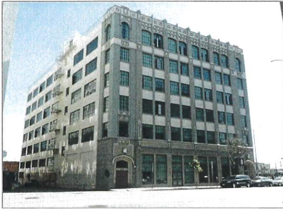
Name: Elias-Katz Shoe Factory Address: 442 S. San Pedro St. Architect: W. Douglas Lee, Florence C. Casler (builder) Date: 1927
