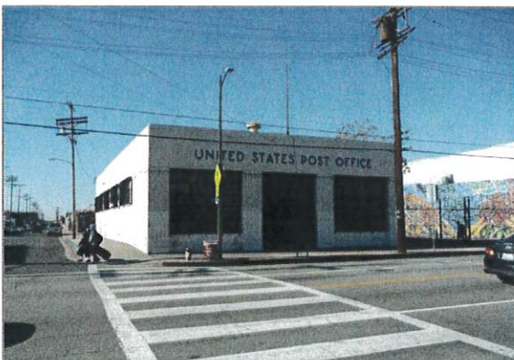
Name: U.S. Post Office, Market Station Branch Address: 1122 E. Seventh St. Architect: John M. Cooper Date: 1940
