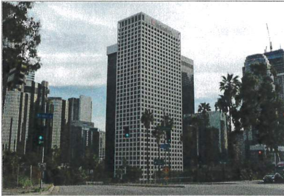
Name: Union Bank Plaza Address: 445 S. Figueroa St. Architect: A.C. Martin and Associates Date: 1966
