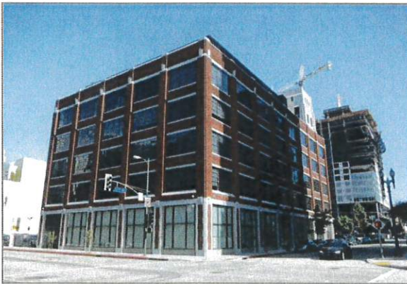
Name: Willys-Knight Building Address: 425 W. Eleventh St. Architect: Morgan, Walls and Morgan Date: 1919
