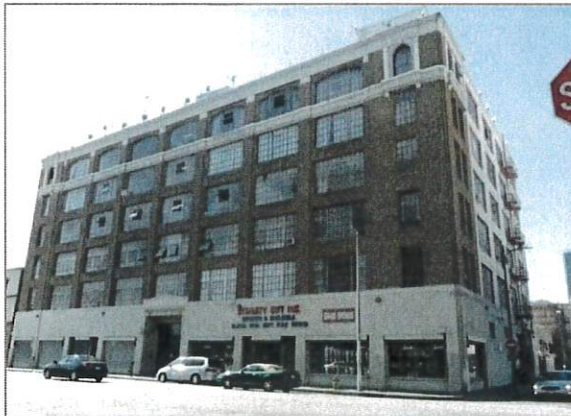
Name: Calo Building Address: 443 S. San Pedro St. Architect: W. Douglas Lee Date: 1923
