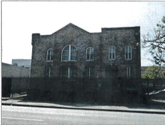
Name: First Free Methodist Church Address: 606 E. Sixth St. Architect: F.A. Brown Date: 1920
