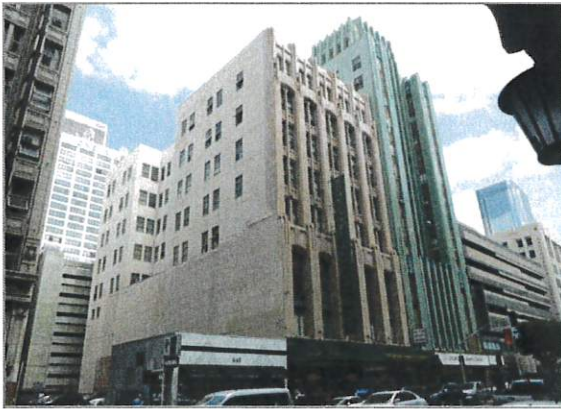
Name: Harris and Frank Building
