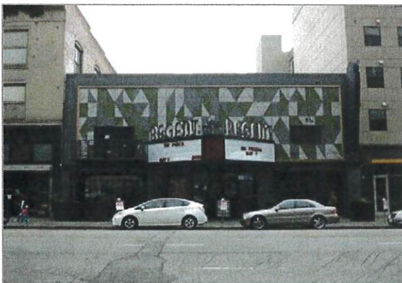
Name: Regent Theatre Address: 448 S. Main St. Architect: A. Lawrence Valk; Stiles Clements (remodel) Date: 1914
