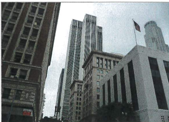
Name: Crocker-Citizens Plaza Address: 611 W. Sixth St. Architect: William L. Pereira and Associates Date: 1967
