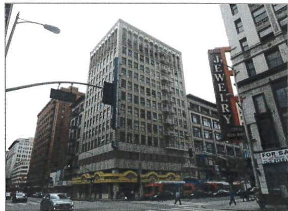
Name: Sun Drug Building Address: 706 S. Hill St. Architect: Curlett and Beelman Date: 1922
