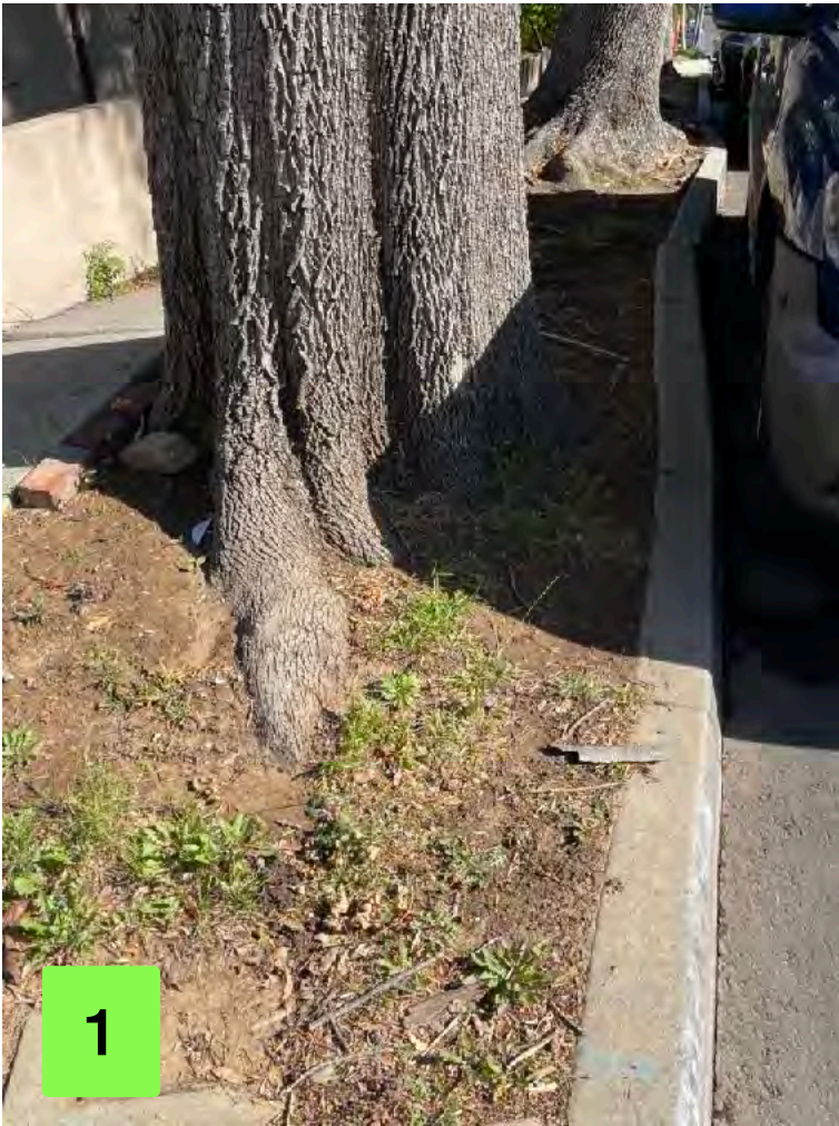
PHOTO 3 - TREE #1 - Raywood Ash ( Fraxinus angustifolia ) street tree #1 damage to sidewalk and curb.
