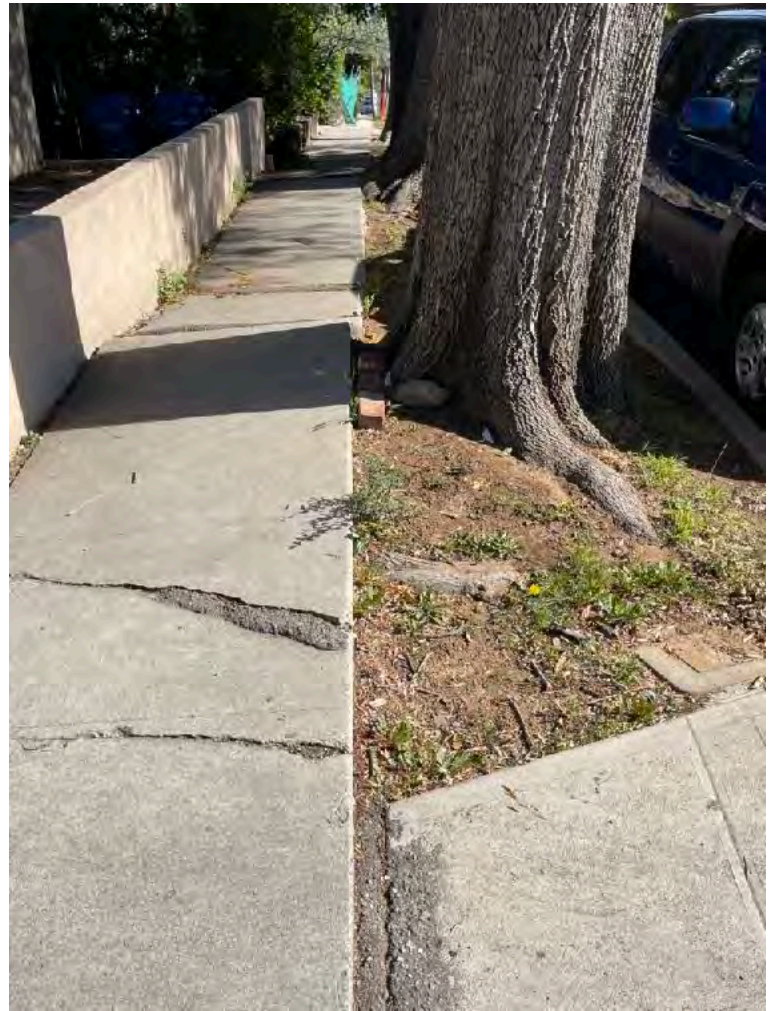
PHOTO 3 - TREE #1 - Raywood Ash ( Fraxinus angustifolia ) street tree #1 damage to sidewalk and curb.
