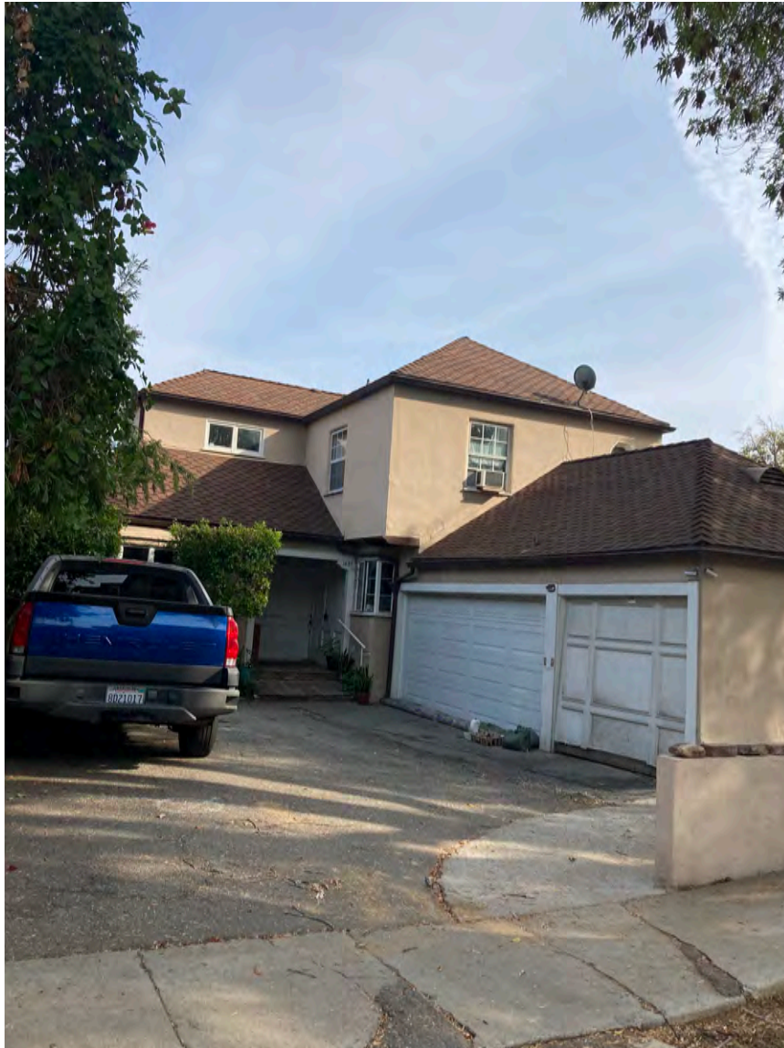
Driveway and entrance to the existing duplex at 1854-1856 S Pandora Ave.
