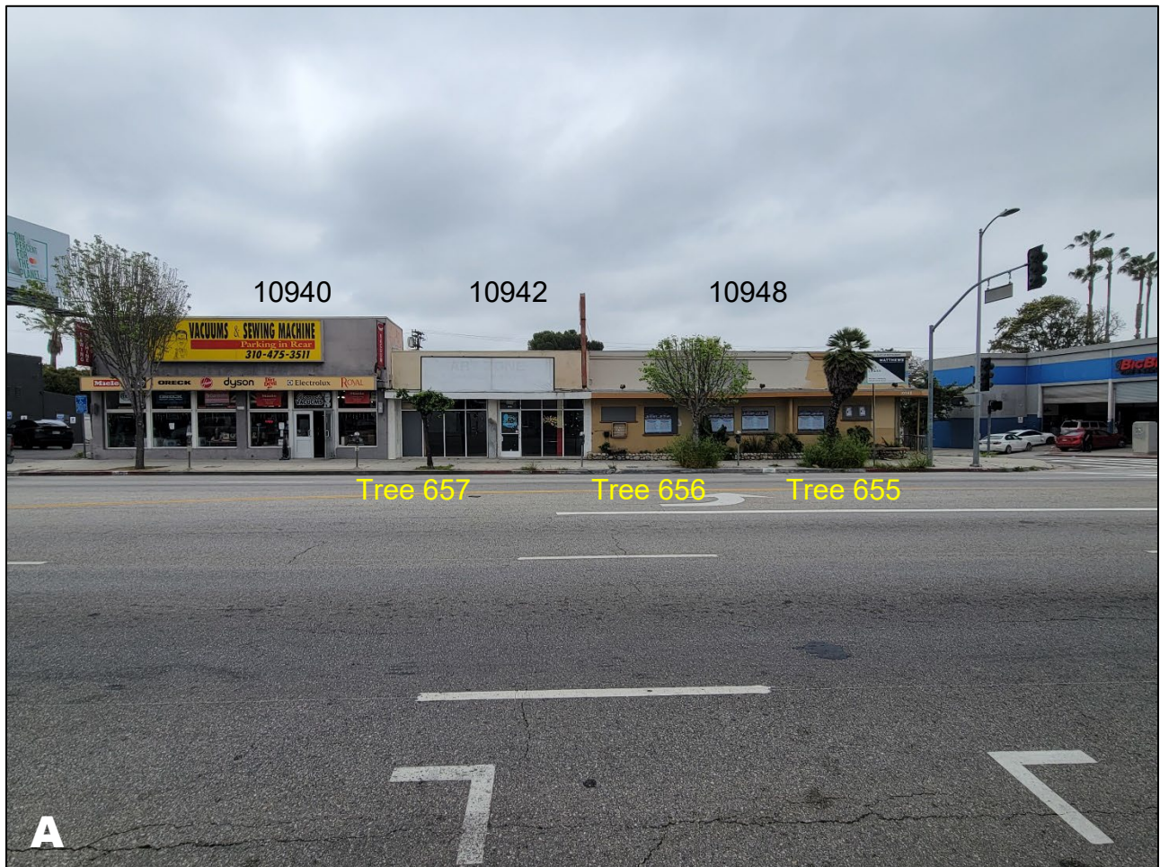
Photo A, facing southeast, showing overview of the 10942 and 10948 W. Pico Boulevard properties and the location of the three City of Los Angeles street trees. The 10940 W. Pico Boulevard property is not part of this development project.
