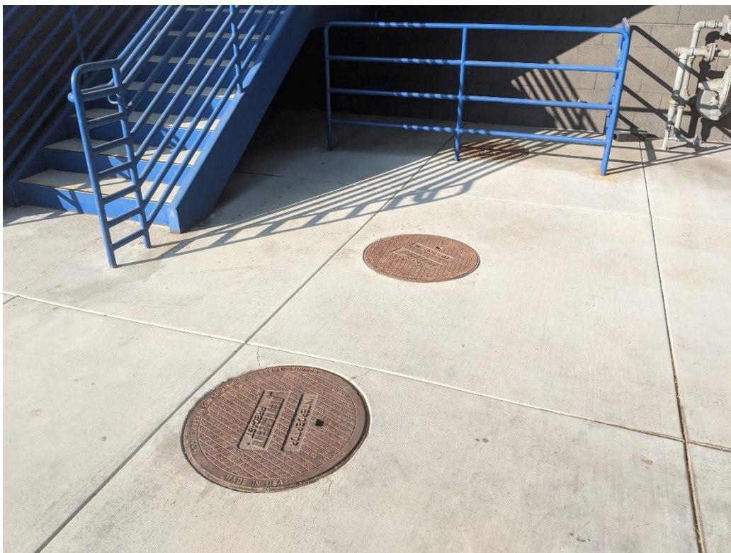
Manholes for the onsite grease interceptor associated with the Chipotle Restaurant. 5240 Lankershim Boulevard, North Hollywood, California 91601
