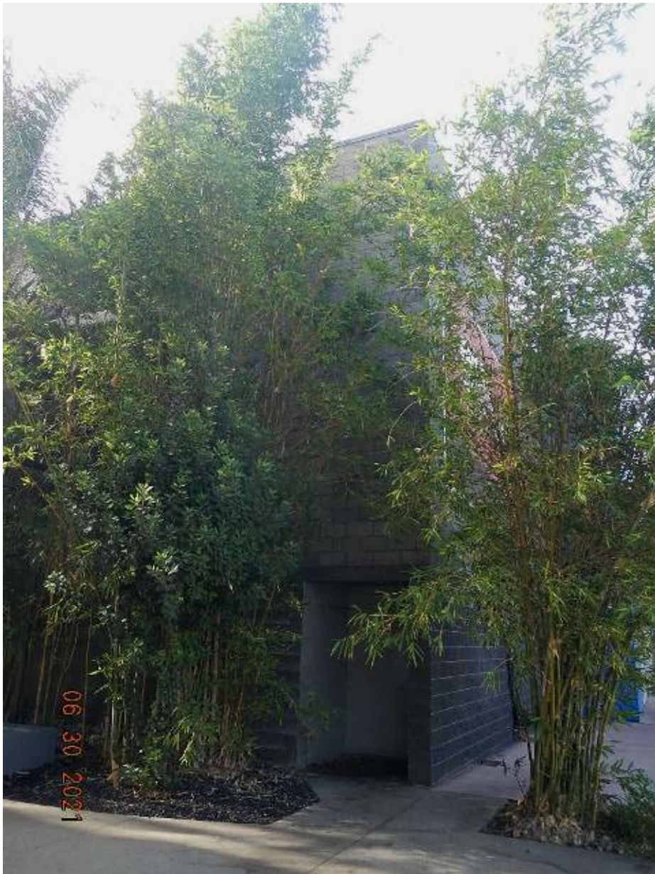
Giant timber bamboo and queen palms run down the north side of the building
