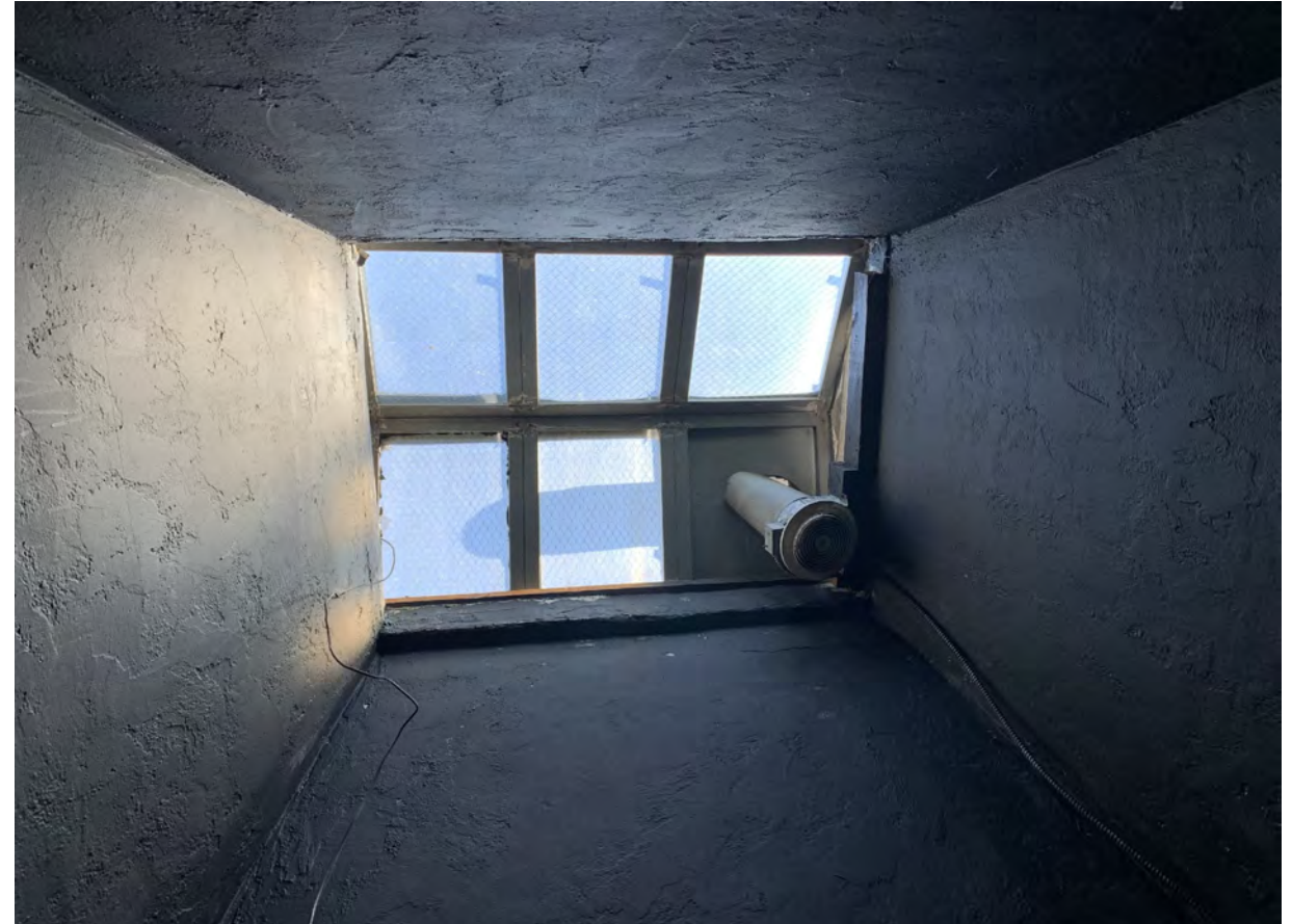
Second floor skylight, 2022. Photo by Lindsay Mulcahy/L.A. Conservancy.
