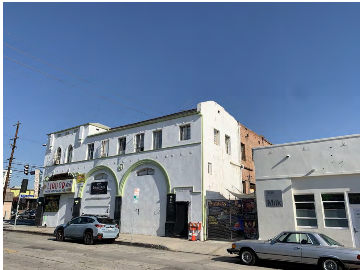
West facade, facing northeast, 2022. Photo by Lindsay Mulcahy/L.A. Conservancy.
