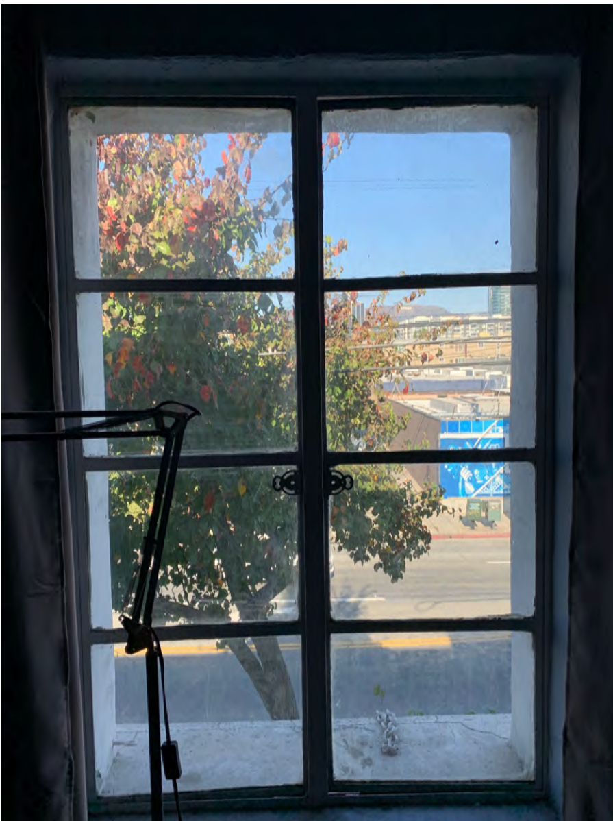
Second story casement window, facing north, 2022. Photo by Lindsay Mulcahy/L.A. Conservancy.
