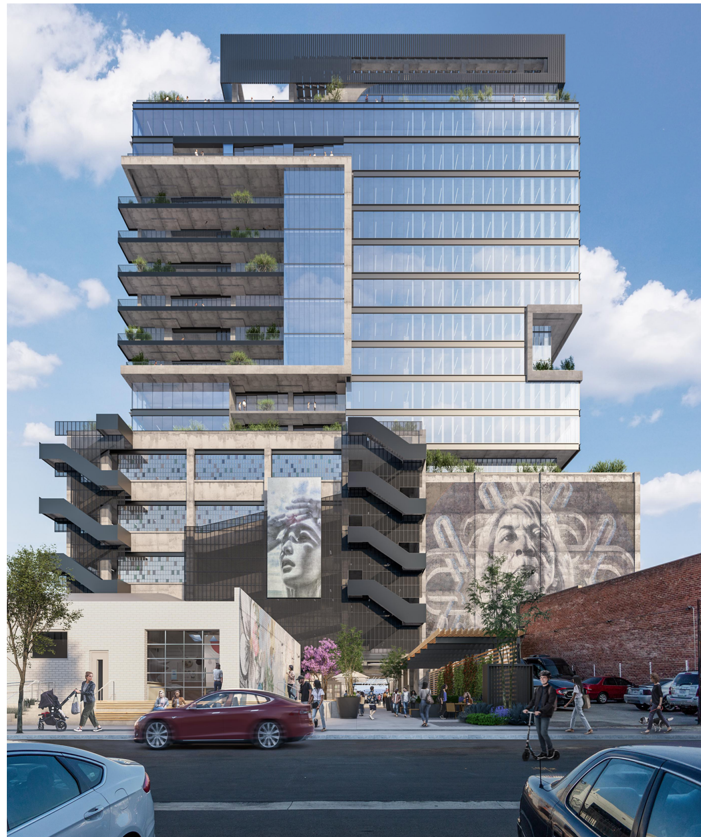
VIEW OF WEST FACADE OF BUILDING
