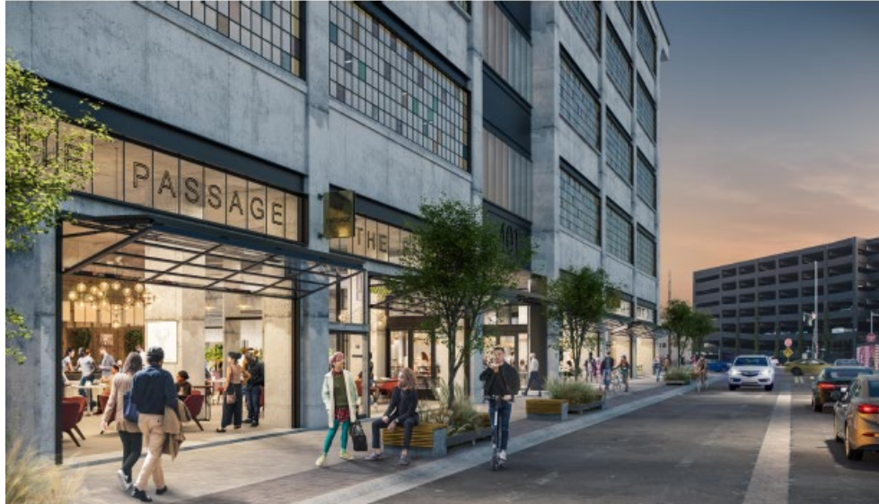
View of Ground Floor Uses and Above Grade Parking Levels along Hewitt Street
