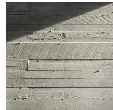
3 EXPOSED CONCRETE W/ FORM-LINER PATTERN
