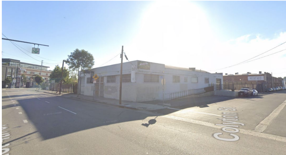
Looking Southeast from 4 th Street at the Bow-Truss Building
