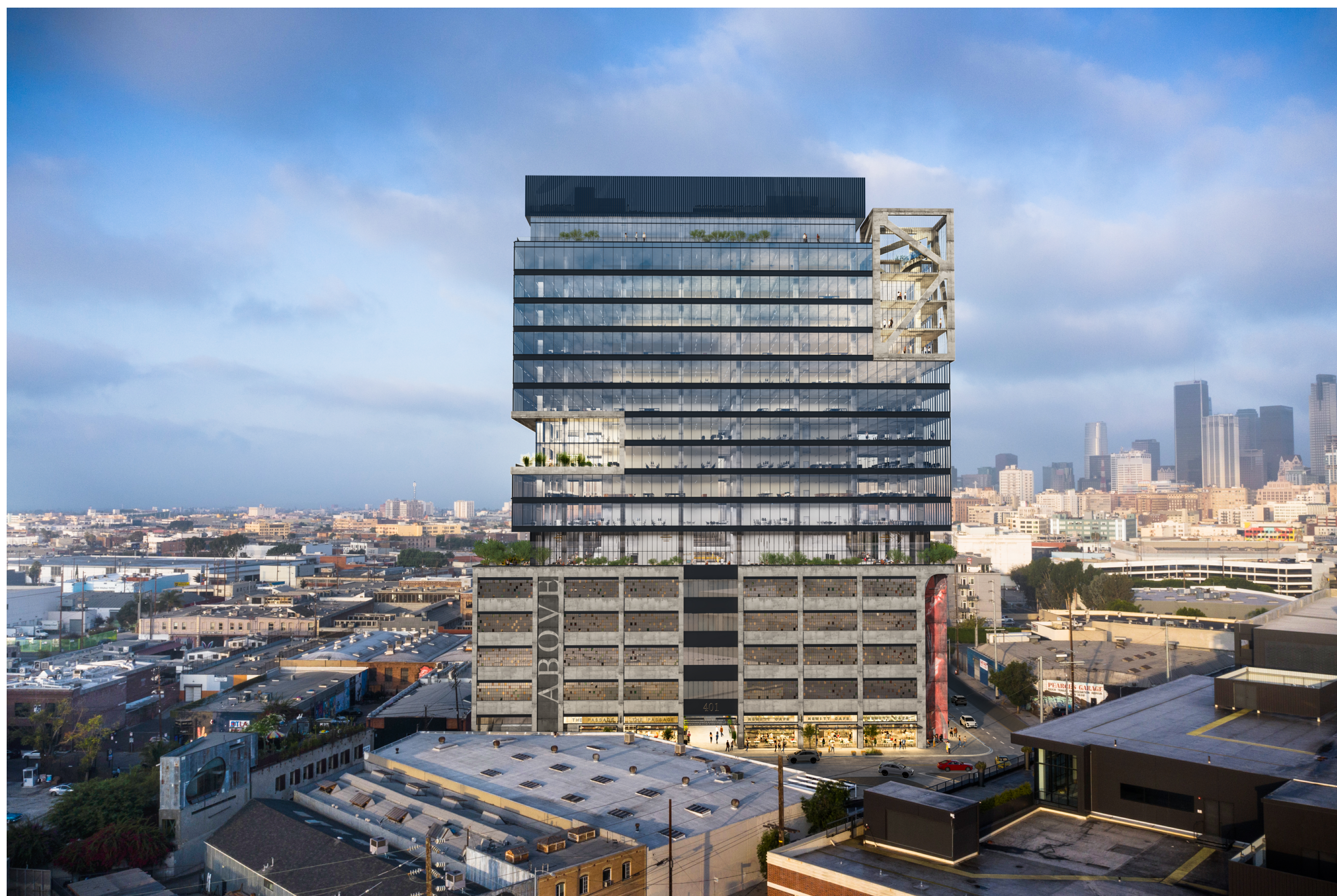
VIEW OF EAST FACADE OF BUILDING
