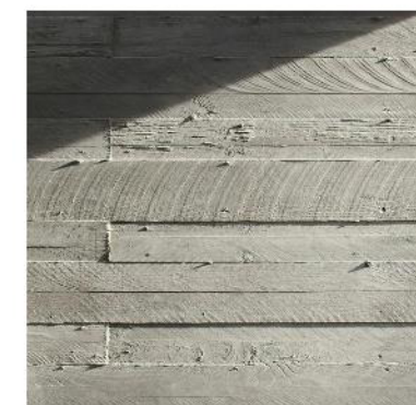
3 EXPOSED CONCRETE W/ FORM-LINER PATTERN
