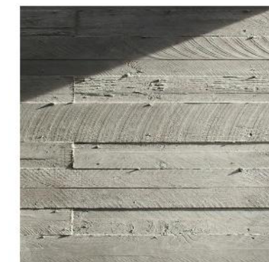
3 EXPOSED CONCRETE W/ FORMLINER PATTERN
