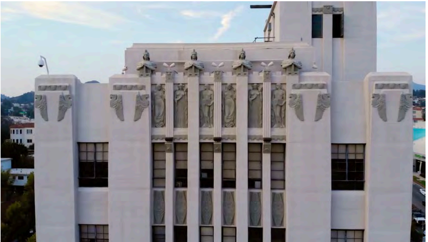
2021: Architectural details of roof (AMDA video tour / Vimeo )
