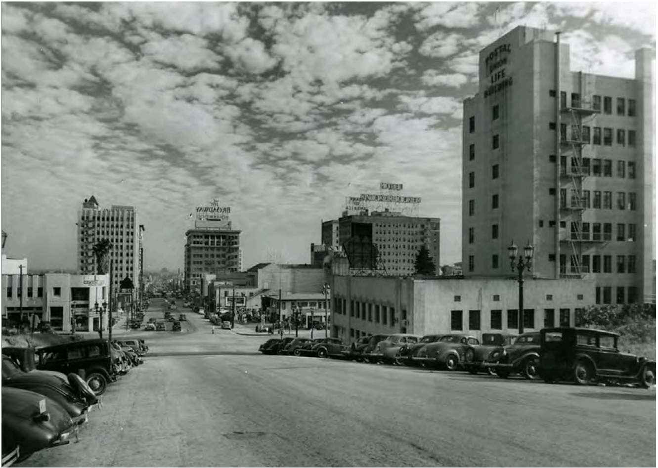
1938: rear/north elevation of the building, looking south on Vine Street (HollywoodPhotographs.com)
