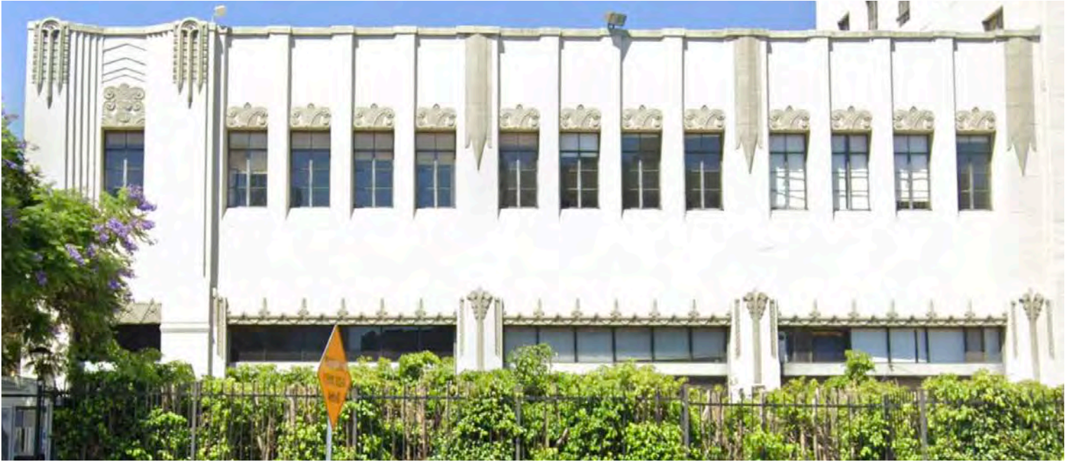
2022: Architectural details of west wing (Google Maps)
