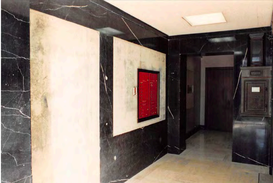
1990s: First-floor lobby, with vinyl wall removed to uncover original marble (photo courtesy of the De Pietro Family)
