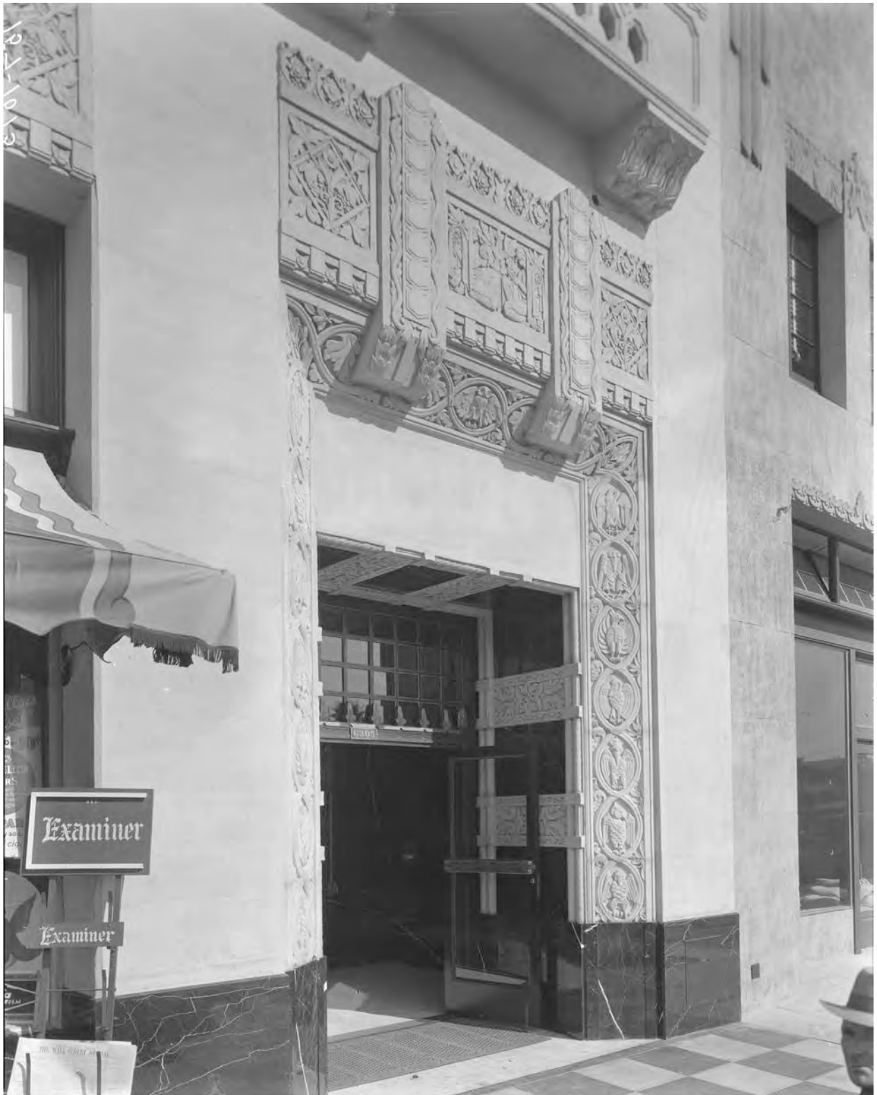
1930: The building's main entrance, framed by bas-relief (California State Library)
