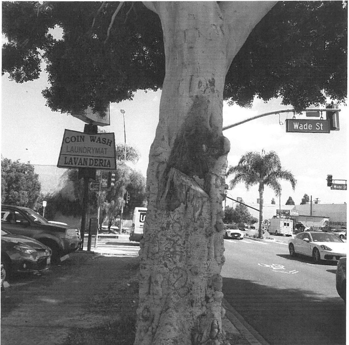
Looking northeast – red arrow indicates old scaffold failure
