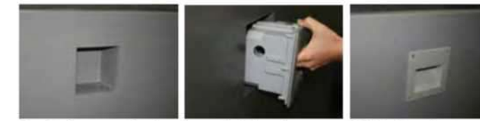
Cast-in Accessory Pocket. Insert light housing. Finished product.
