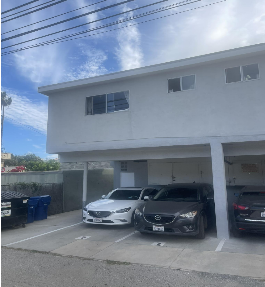
2) Photo of the neighboring property from the alley
