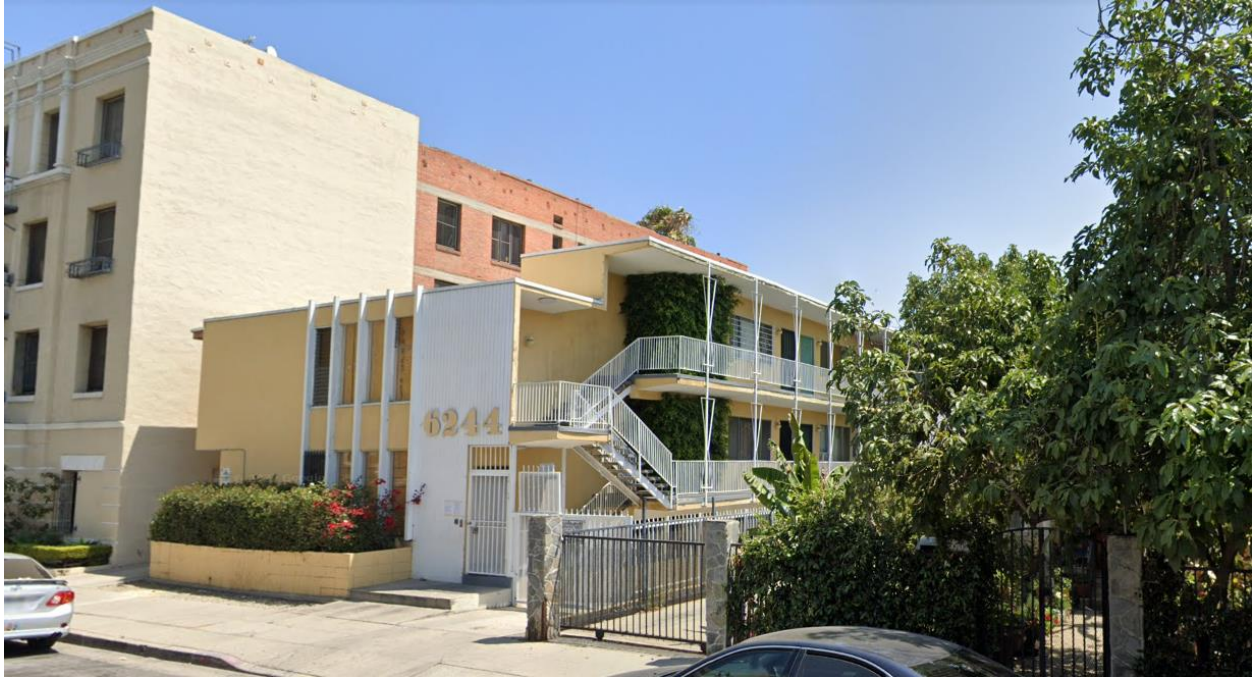
Figure 1: Breezeway at residential building near Residential Receptor R2.
