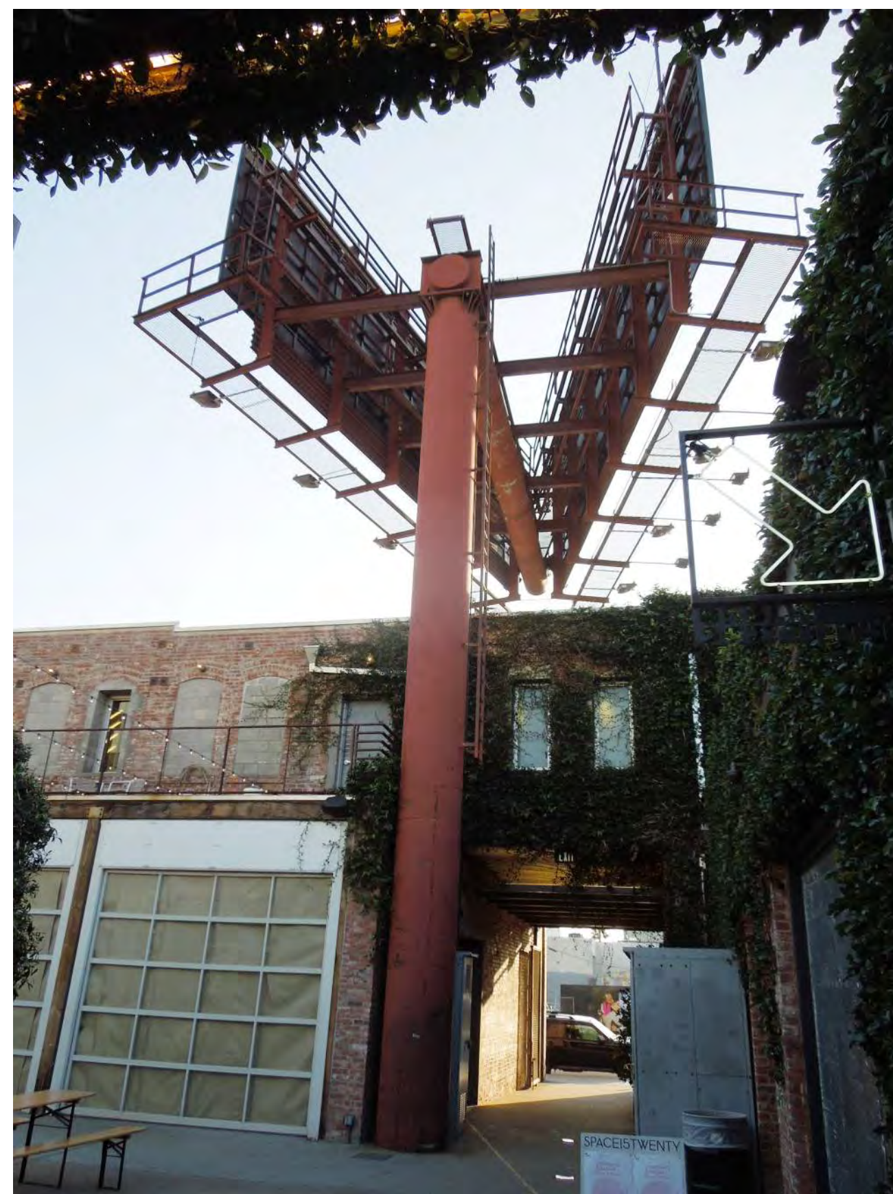
05 EXISTING COURTYARD FOR "SPACE 15 TWENTY"
