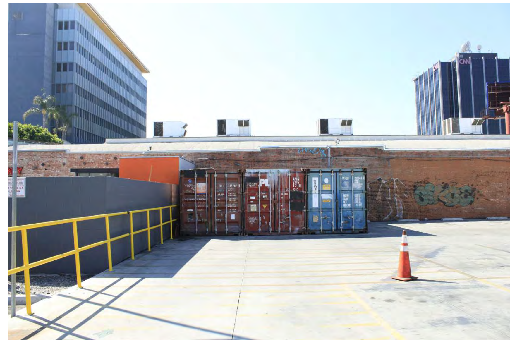
02 VIEW AROUND THE EDGE CONDITIONS OF THE EXISTING SURFACE PARKING LOT
