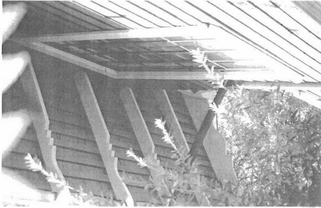
South elevation: Second level shaped eave corbels, paired multi-pane French doors, viewed to west.
