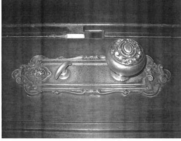
Front door hardware detail, interior, showing elaborate cast brass escutcheon and door knob with lion depicted in relief.
