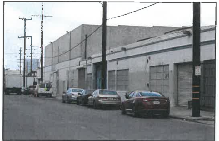
View 2: From the south side of Industrial Street looking northwest at the Project Site.
