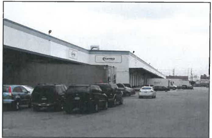
View 8: From the north side of Wholesale Street looking north-east.
