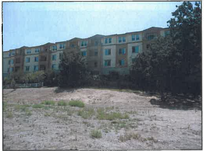
Photo F: View toward the south of the multi-family residential building located adjacent to the western portion of the Project site.
