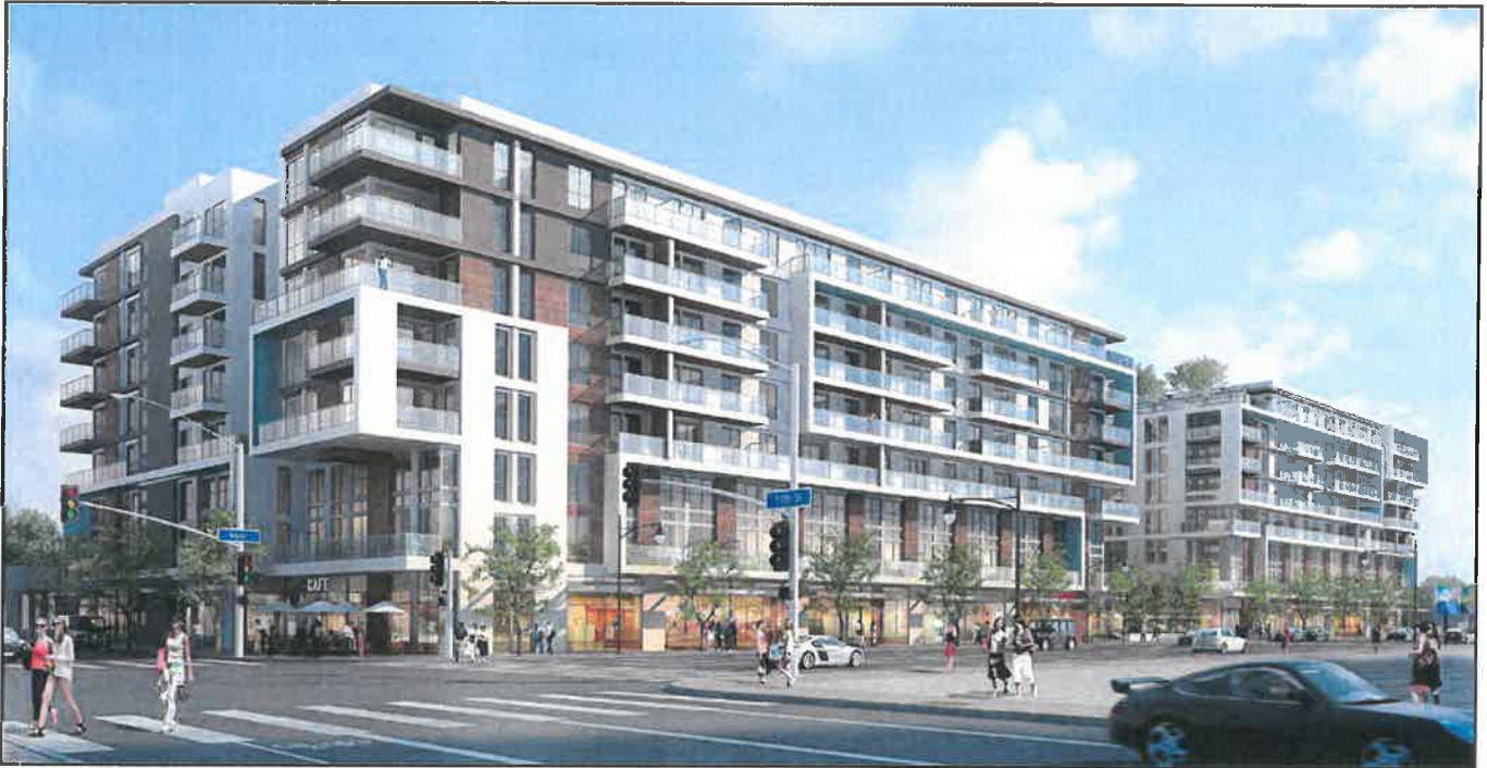
View of Proposed Project from Main Street and 11th Street.
